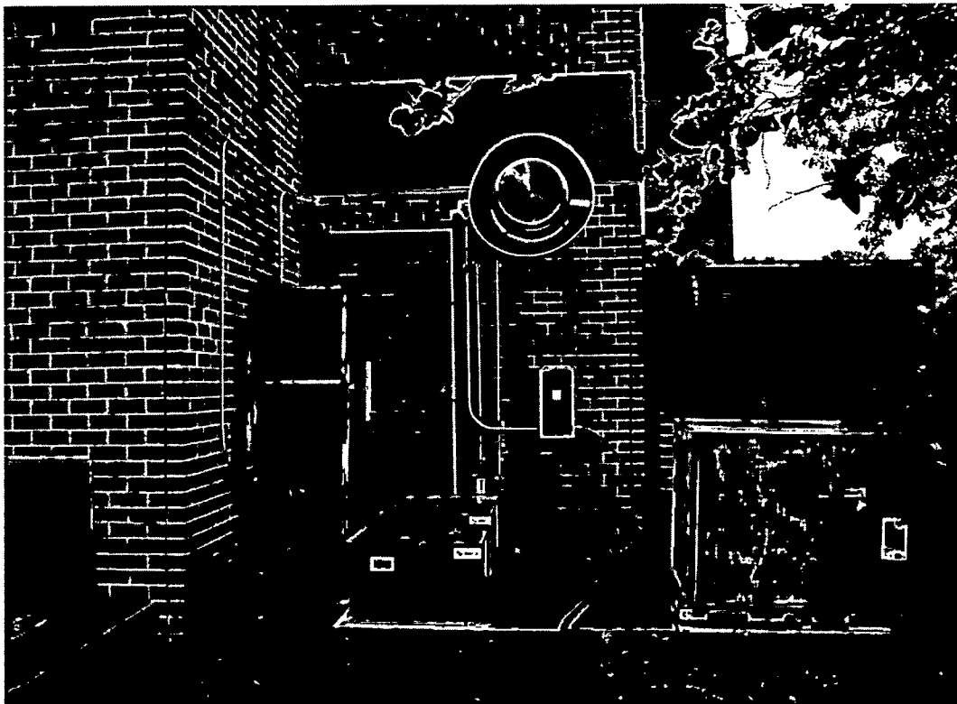
7051 Carroll Ave. East Elevation view of exhaust fan to be removed.
