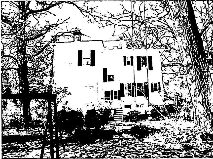
View of Existing Rear Façade
