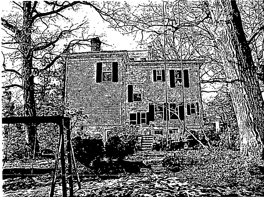
View of Existing Rear Façade
