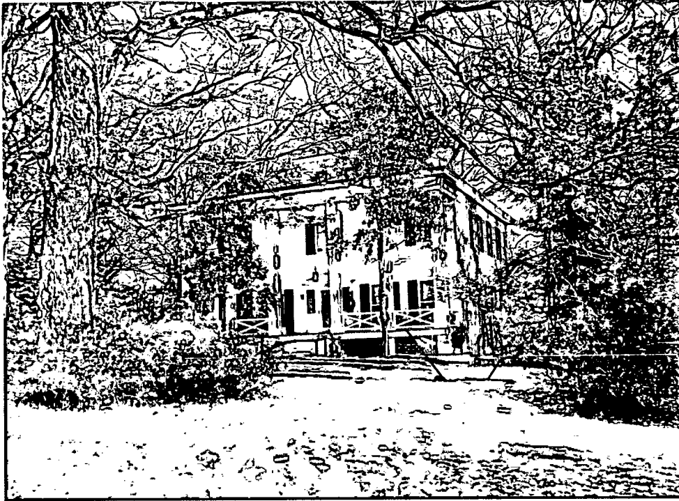
View of Front Façade from Buffalo Avenue. No Change Intended.
