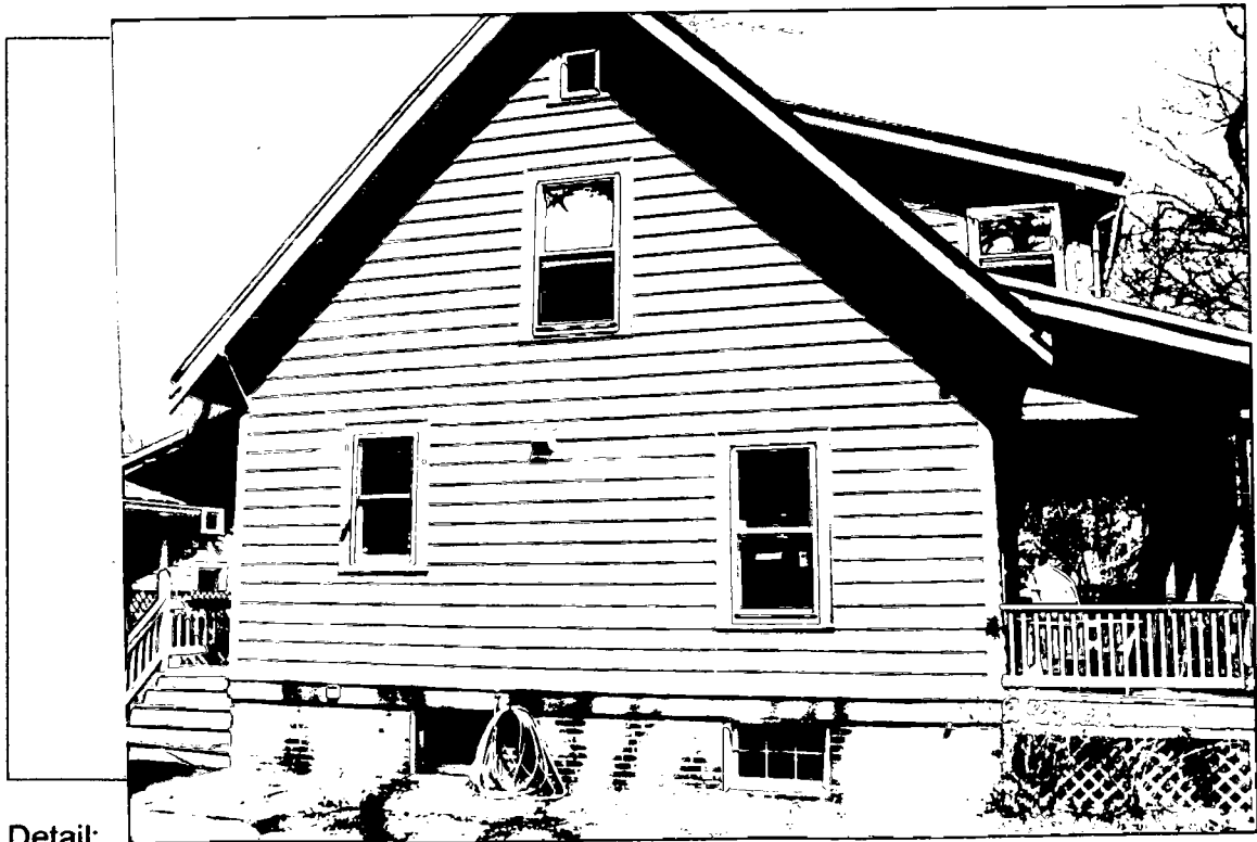
Detail: view from South Downer visible upper left
