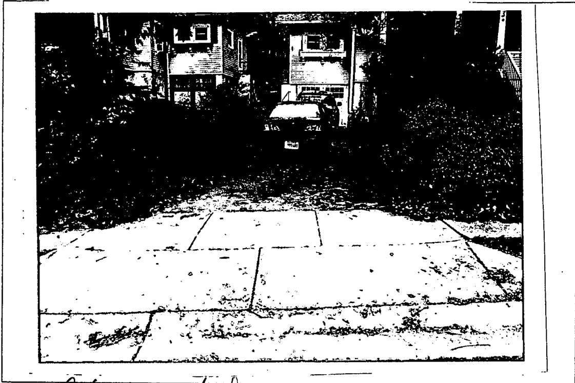
Detail: Close up of the existing driveway & apron
