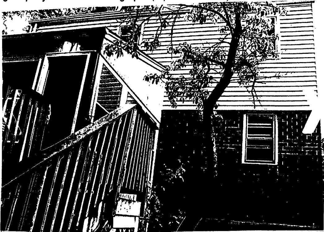
Detail: Rear of 13 Columbia (unaffected by this project)
