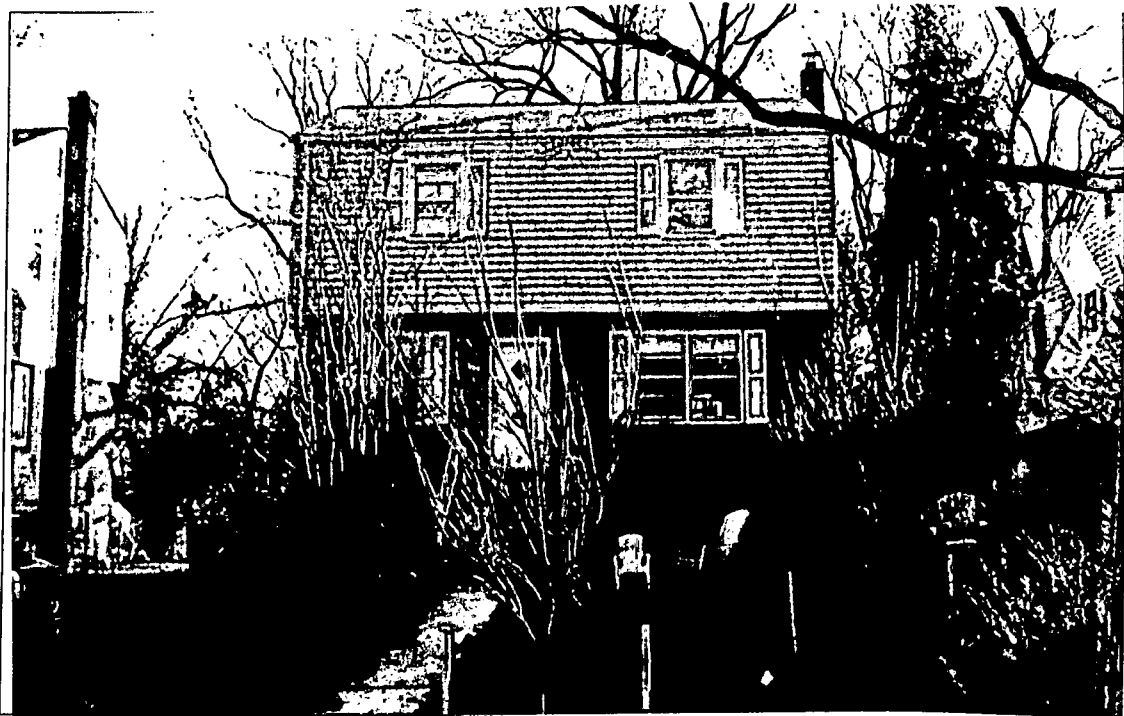
Detail: Front of 13 Columbia from street.
