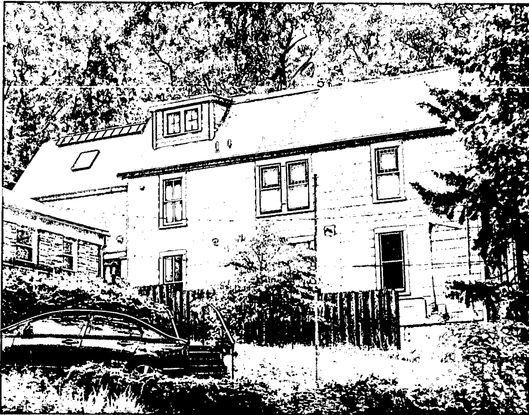
Detail: View from north side
