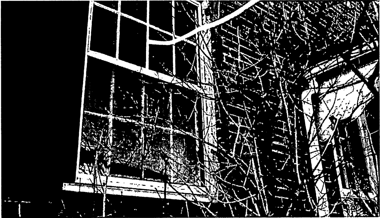
DETAIL: shutters to be removed to match opposite side of house which doesn't have shutters
