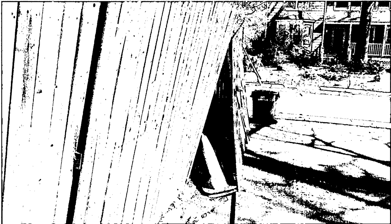
DETAIL: BROKEN FENCE – VIEW FROM CARPORT
