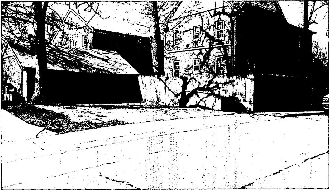
DETAIL: BROKEN FENCE – VIEW FROM across the street - new fence will enclose half the carport
