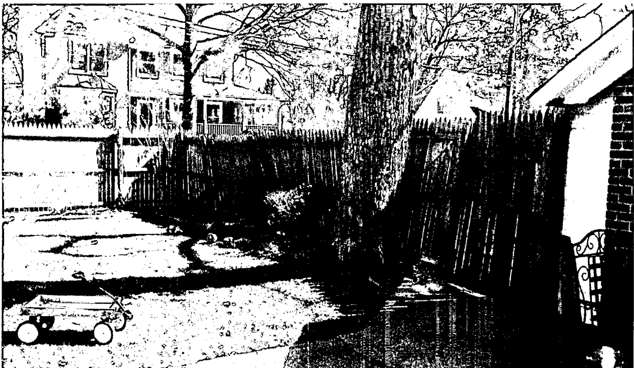
DETAIL: Broken fence – view from back yard
