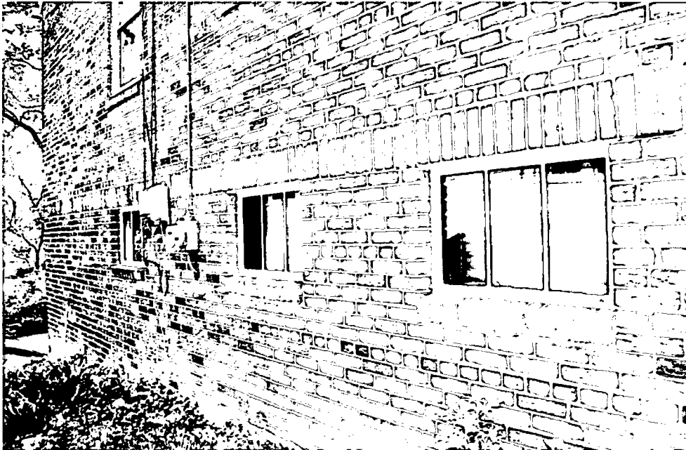
Driveway side of house. 3 casement windows.
