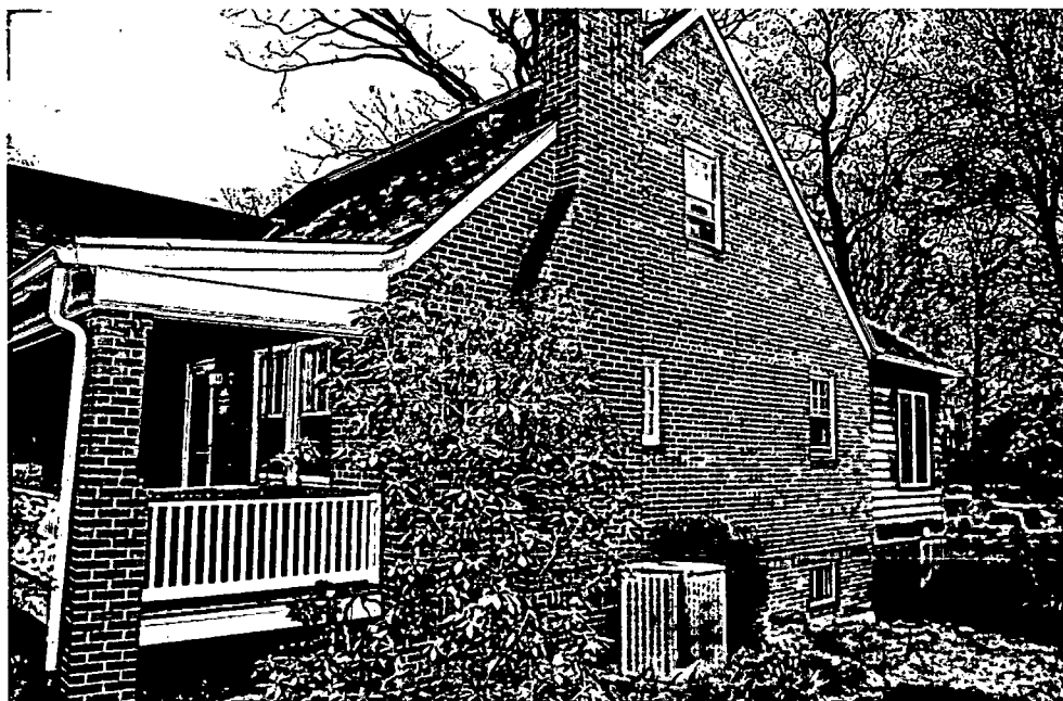
Northwest side of house, 2 casement windows
