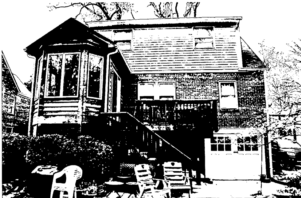
Rear of house, no casement windows.
