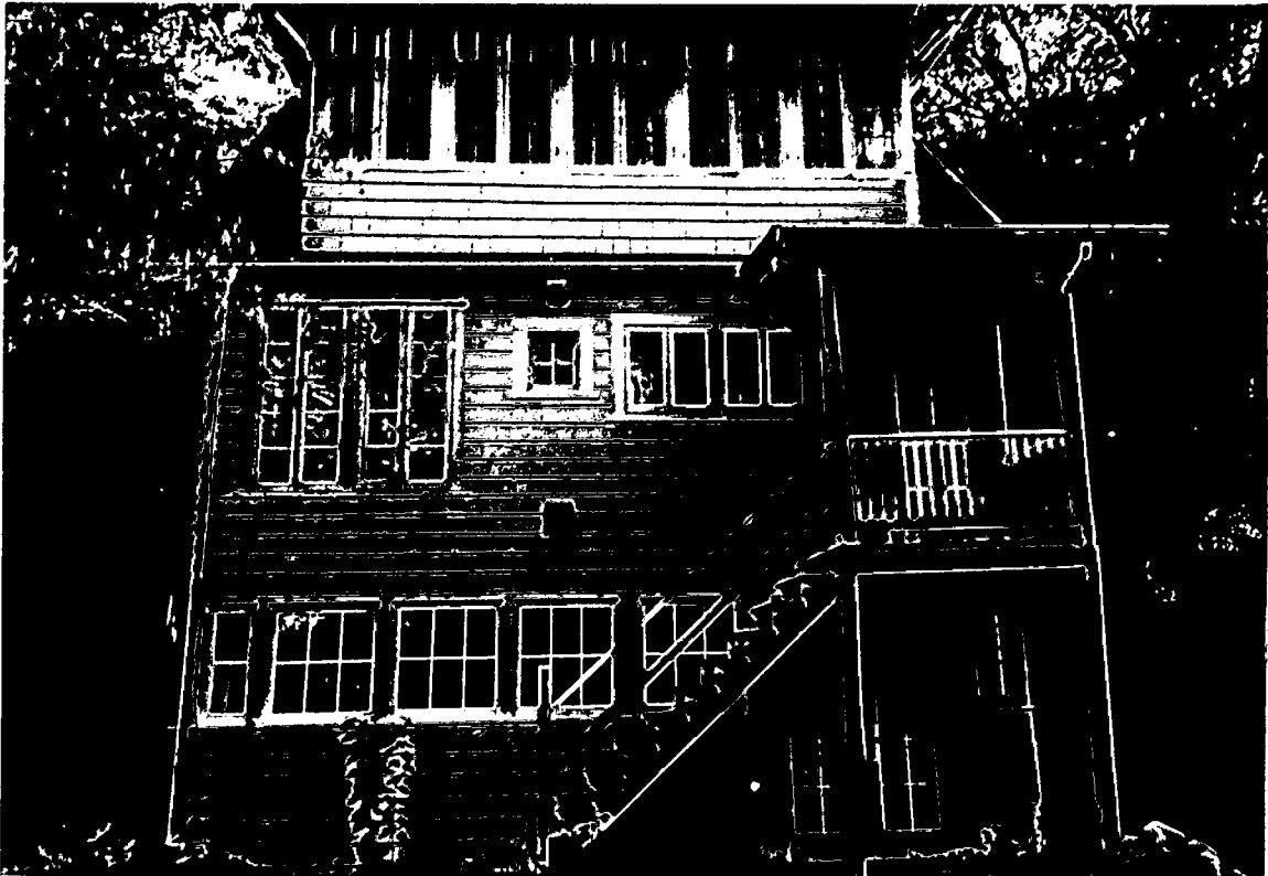
Detail: Back of house, back yard, deck and stairs to be taken down / replaced
