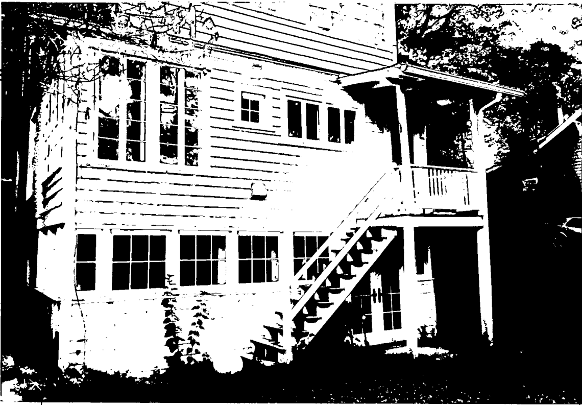
Back of house - deck taken from western angle - direction of Westmoreland Ave.
