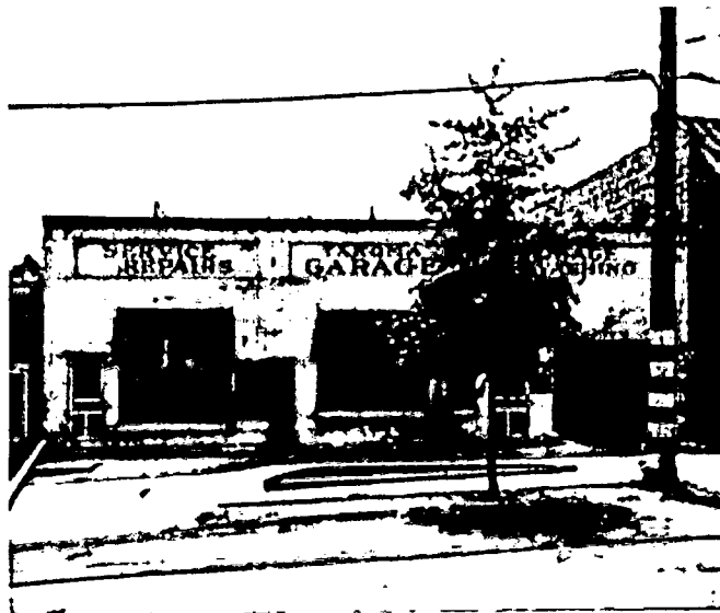
Original Garage Prior to 1941
