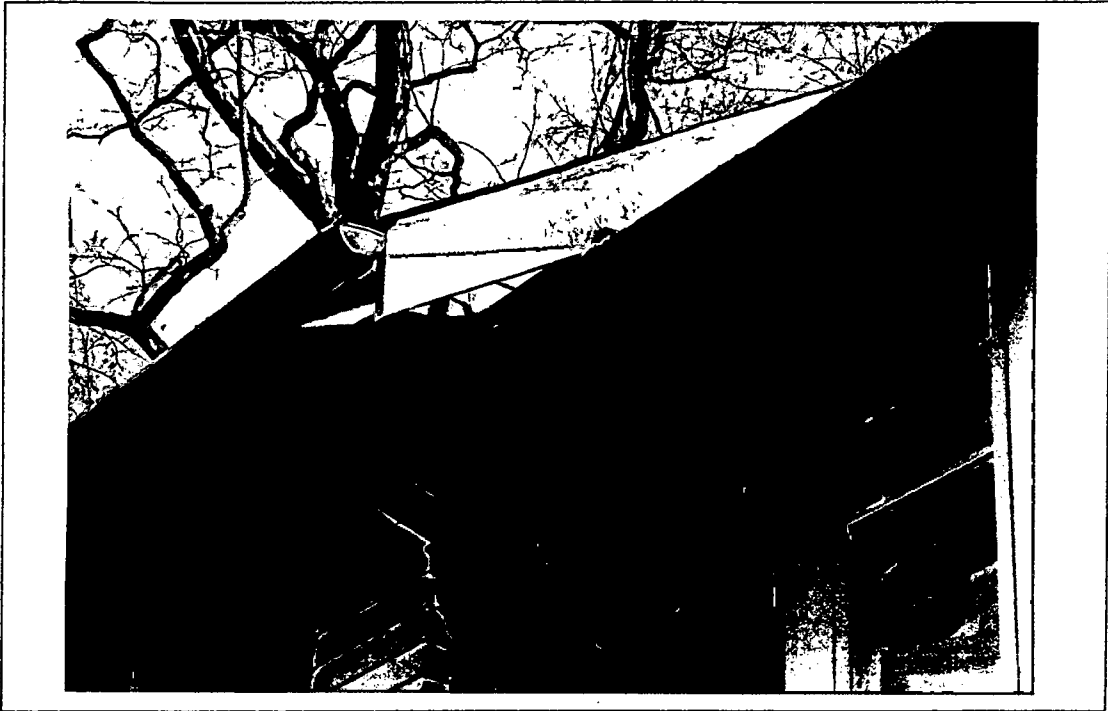
Detail: COPPER GUTTERS & DOWNSPOUTS
