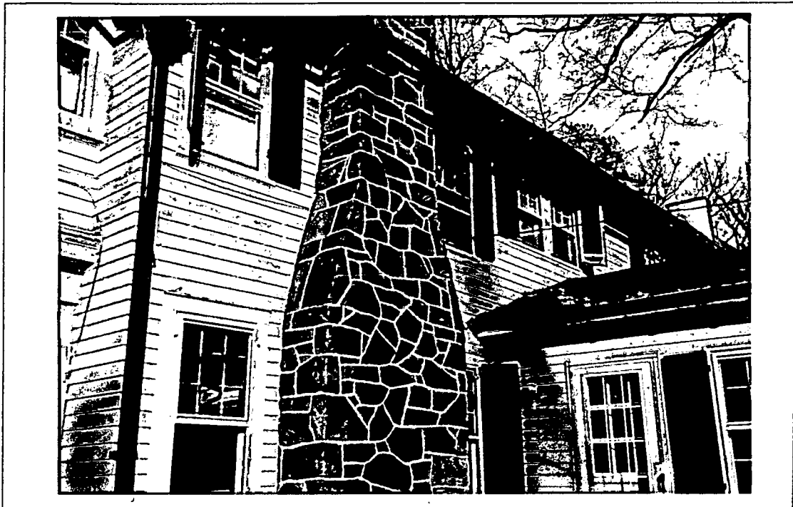
Detail: STONE CHIMNEY
