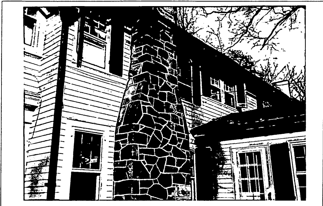
Detail: STONE CHIMNEY
