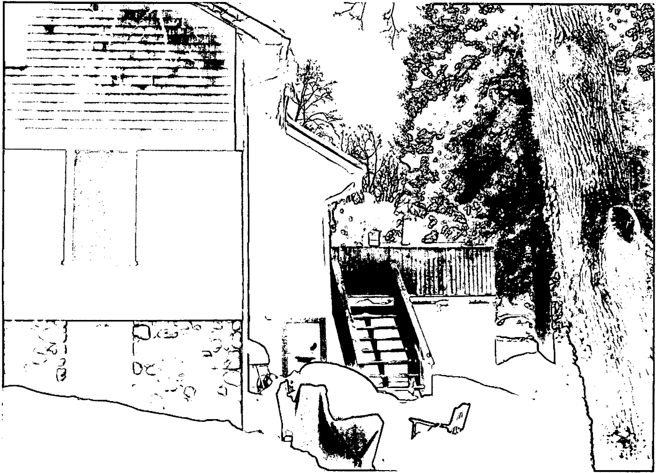
REAR CORNER, GARAGE, + STAIRS
