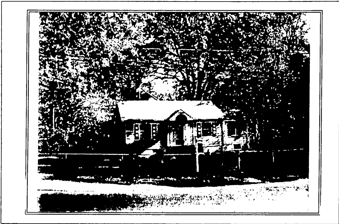
Detail: Front view of property with chain link fence
