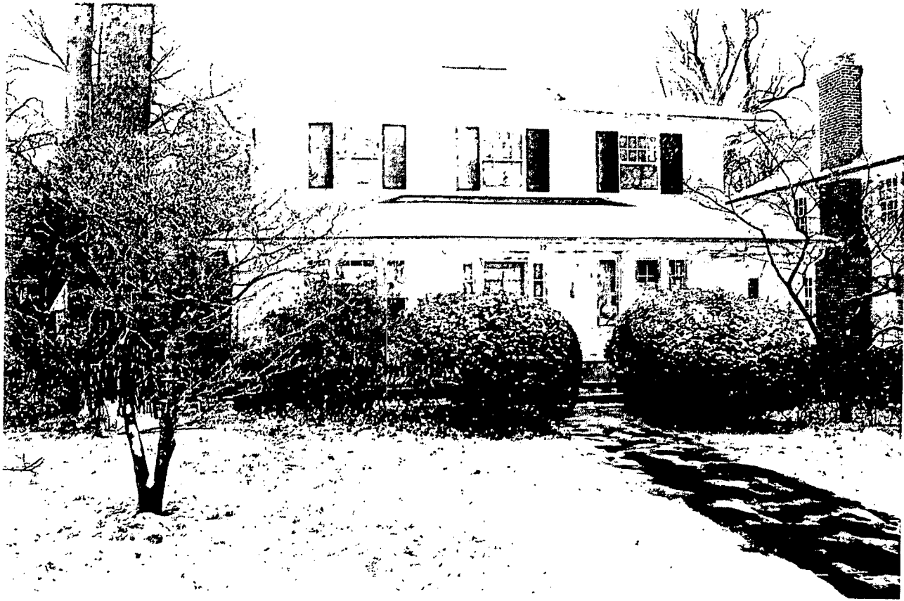
Existing Front Elevation of 22 W. Irving (View from ROW)
