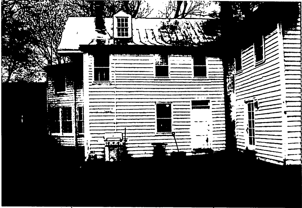
DETAIL - REAR ELEVATION OF INSIDE CORNER ADDITION SEE SEE PROPOSED ELEVATIONS FOR CHANGES
