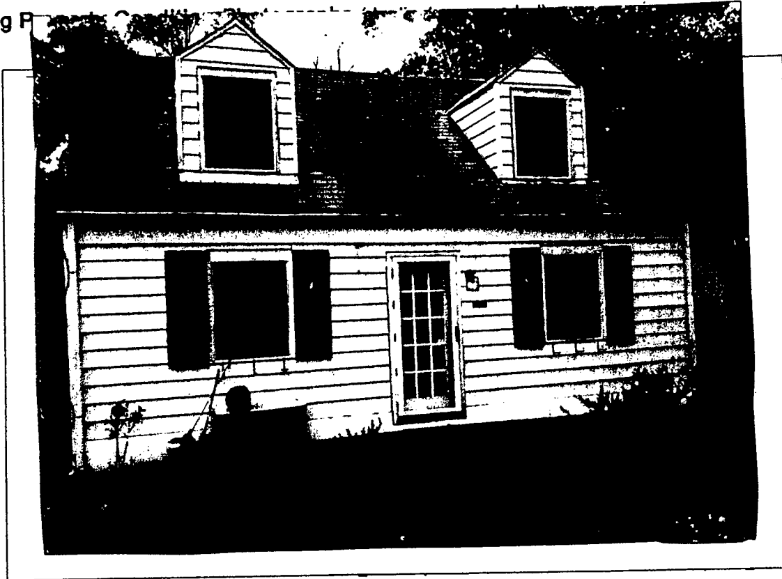
Detail: House front
