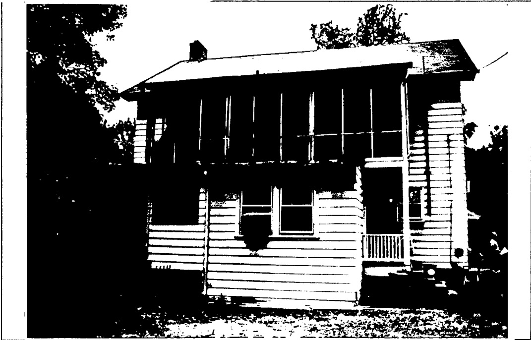
Detail: REAR ELEVATION - FACING SOUTH (#4 HESKETH ST.)
