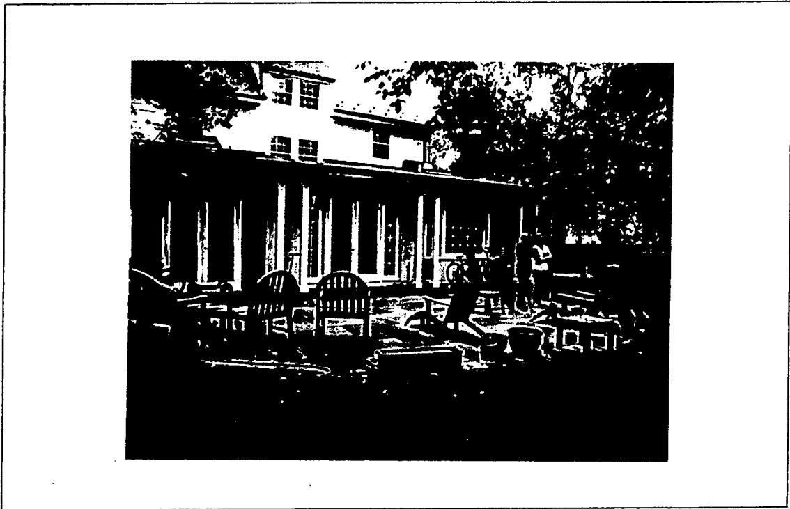
Detail: 7 Hesketh Street, existing condition
