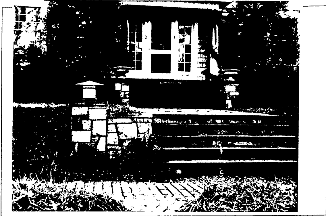
Detail: 8 West Irving, model for stone stairs with pillars, (but mortar will be recessed instead)
