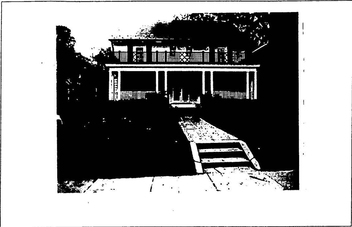
Detail: 7 Hesketh Street, existing condition
