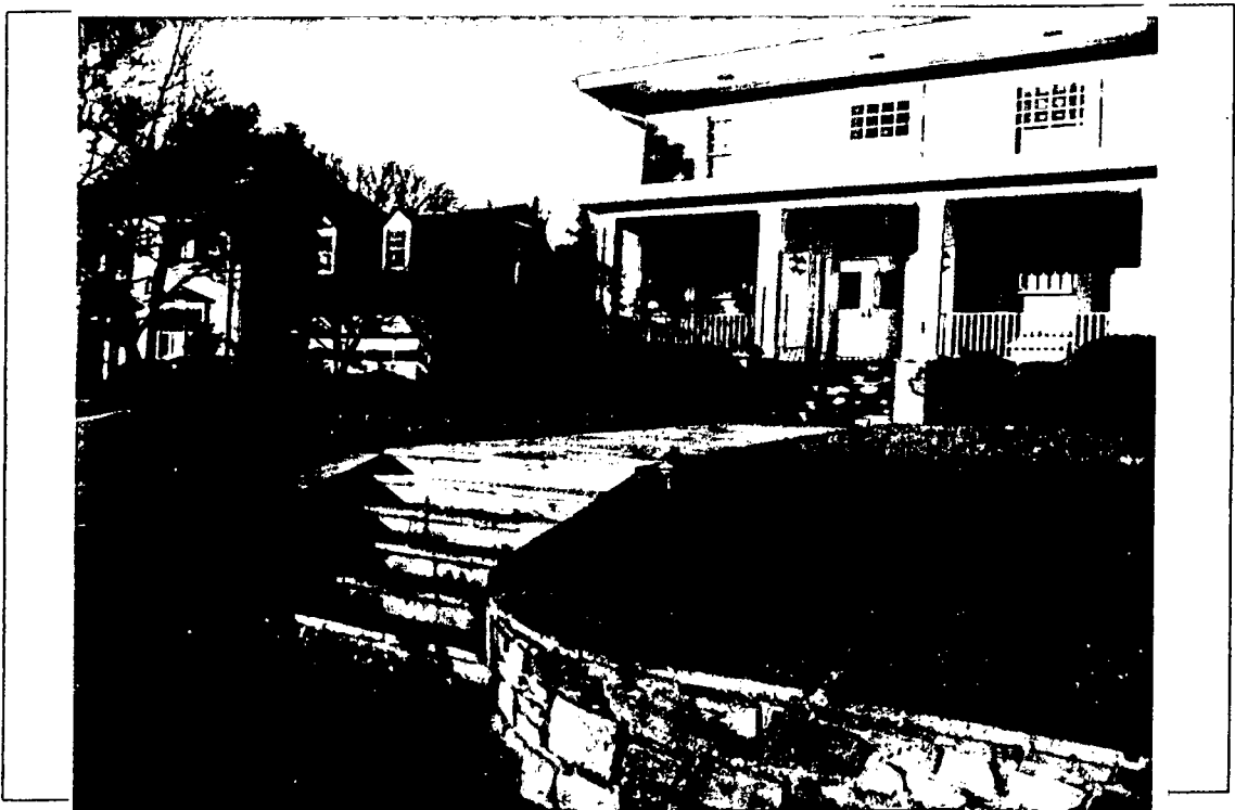
Detail: 15 Grafton, shows retaining wall at edge of sidewalk (intend to build)
