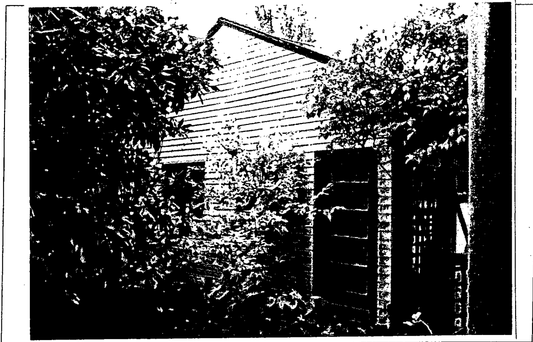
Detail: LEFT SIDE OF GARAGE
