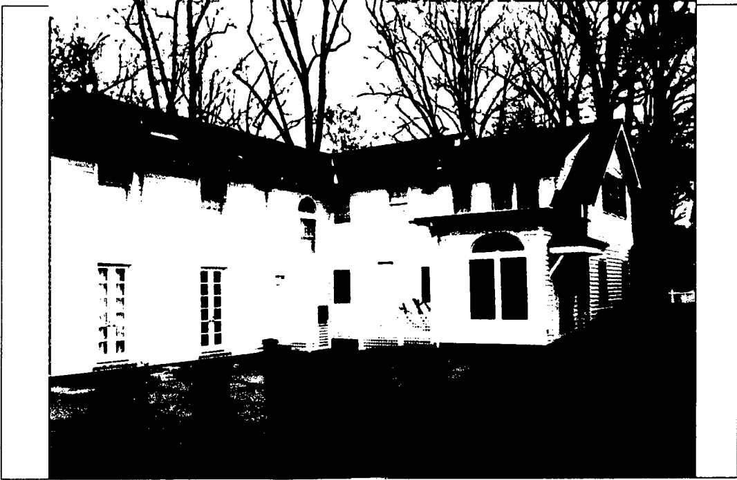
Detail: Rear view of South and West elevations
