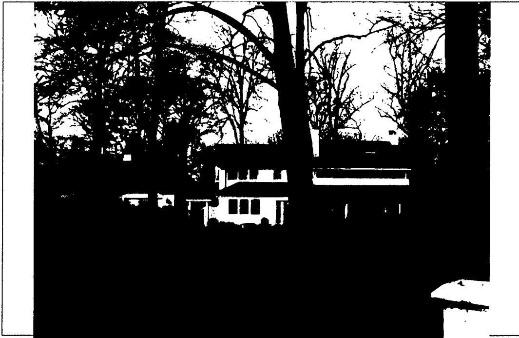
Detail: East Elevation view from Magnolia Street
