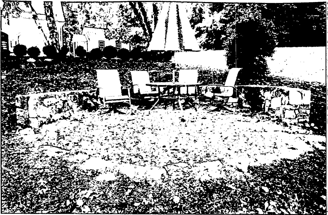
Detail: Pea Gravel Base on patio is deteriorated. Replacing w/ matching slate.
