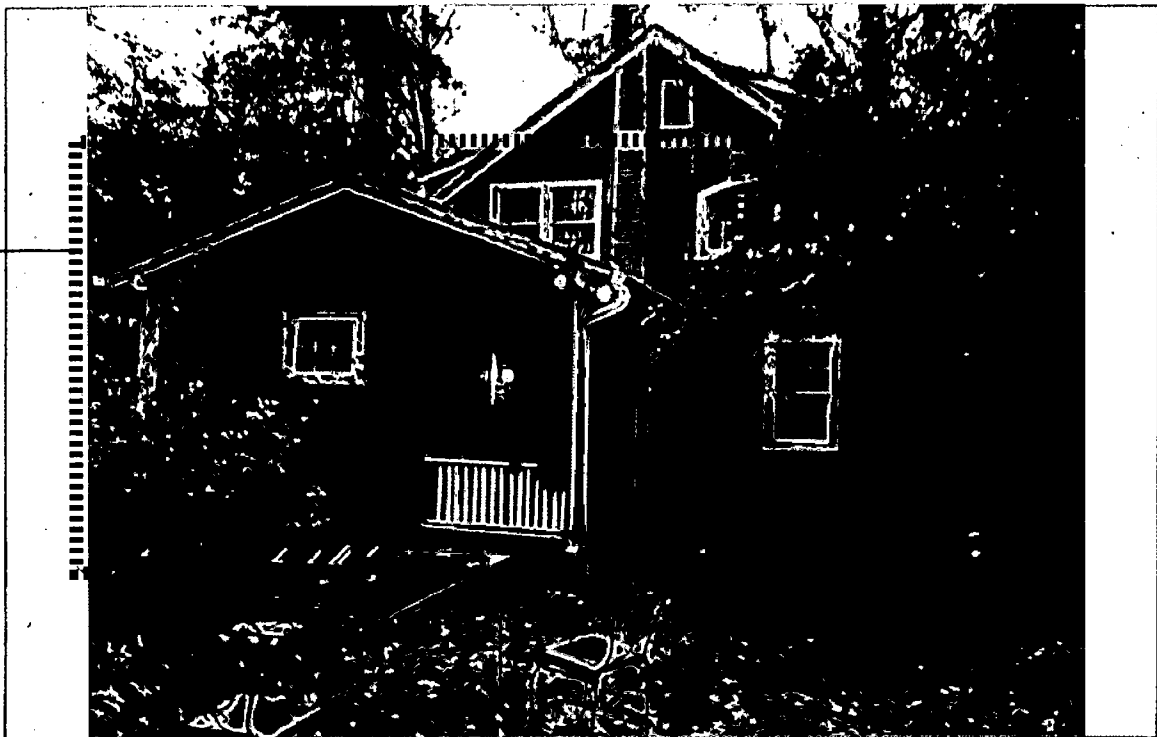
Detail: South Facade (Rear Yard)
