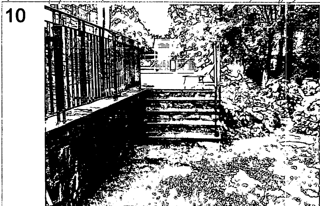
Detail: View Towards lowest set of steps from pool deck (area of future guardrail + 1 additional step)
