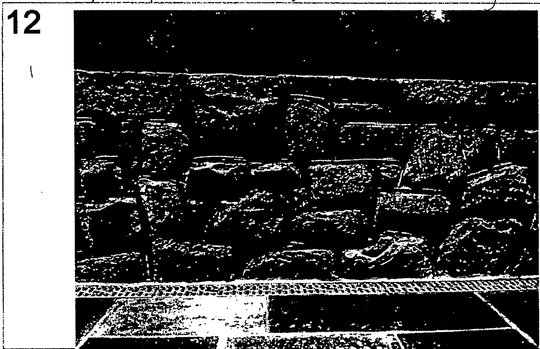
Detail: View towards existing wall (part of wall to be replaced with railing)
