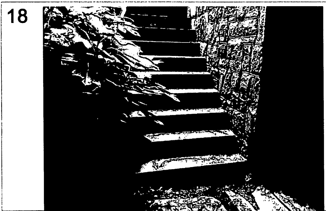
Detail: View Towards steps leading to lower level pool storage area below pergola (Area of future gates and fencing)
