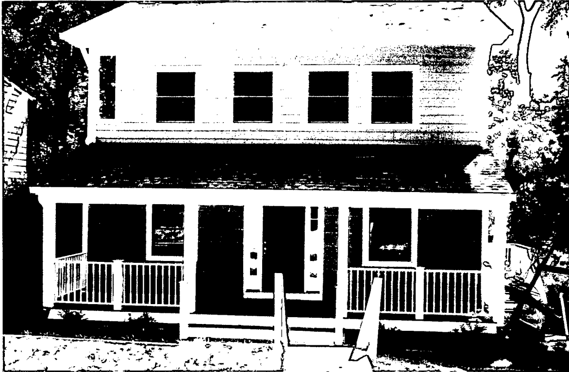
ADJACENT PROPERTY TO NORTH (FRONT)
