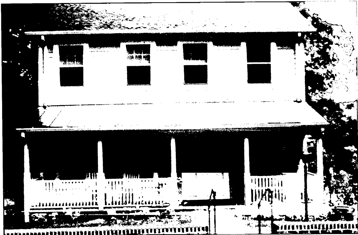
FRONT/WEST ELEVATION, SUBJECT PROPERTY
