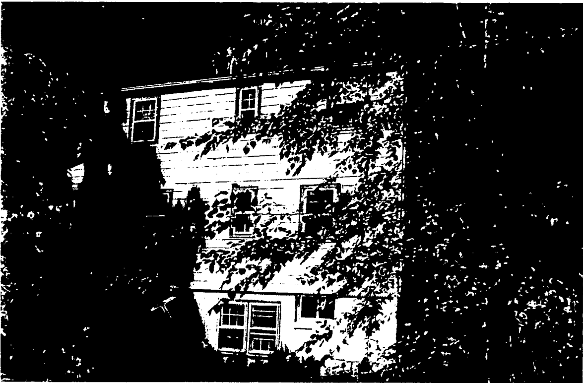
ADJACENT PROPERTY TO SOUTH (REAR)
