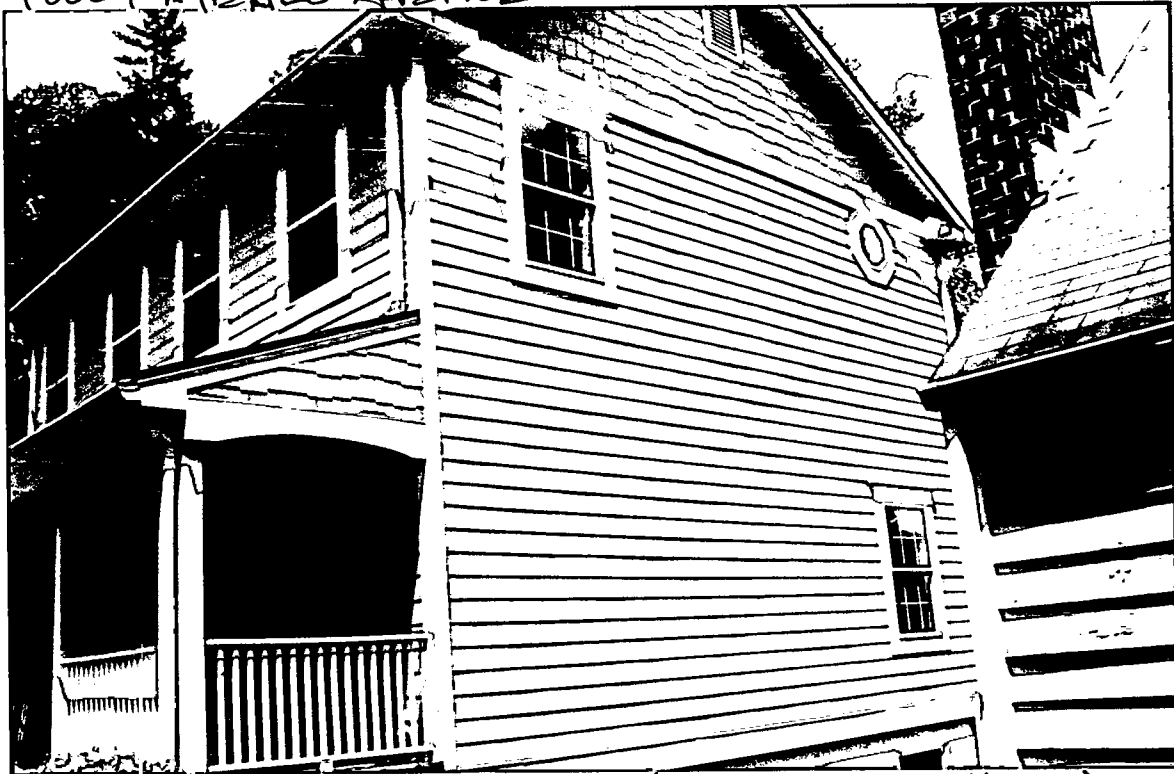
RIGHT/SOUTH ELEVATION (FROM FRONT OF HOUSE), SUBJECT PROPERTY
