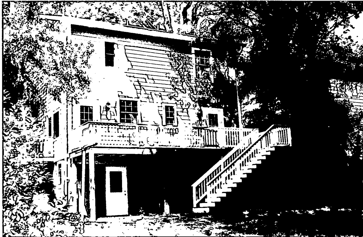
ADJACENT PROPERTY TO NORTH (REAR)
