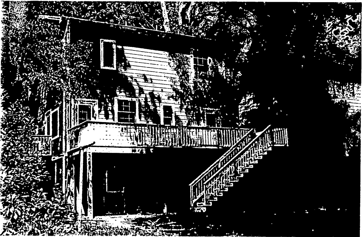
ADJACENT PROPERTY TO NORTH (REAR)
