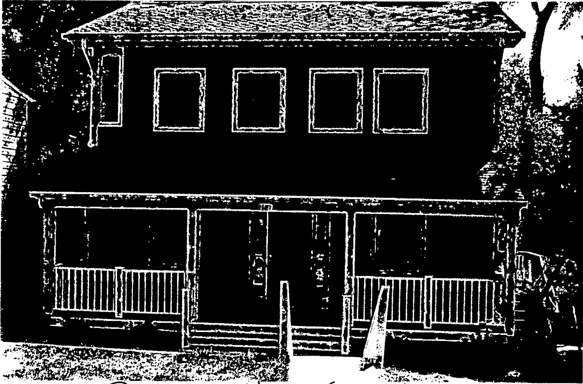
ADJACENT PROPERTY TO NORTH (FRONT)
