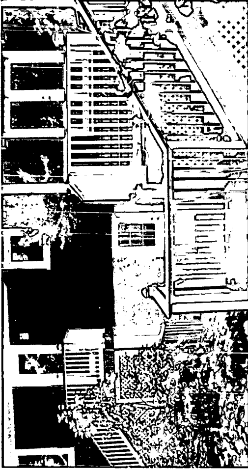
Location of new deck (above basement door) connecting existing mudroom landing (on left) with existing deck (on right). Stair in foreground to be removed.
