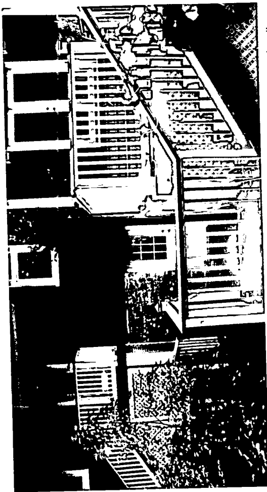
Location of new deck (above basement door) connecting existing mudroom landing (on left) with existing deck (on right). Stair in foreground to be removed.
