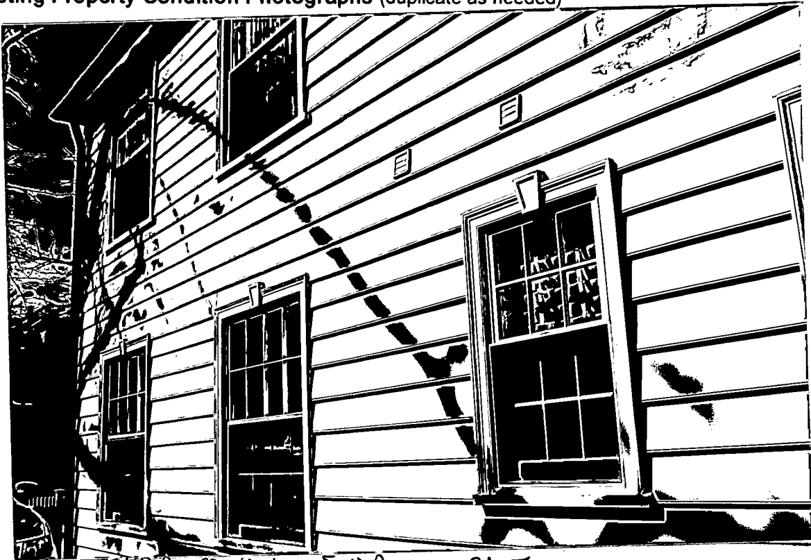
Detail: B DRIVEWAY SIDE EAST
