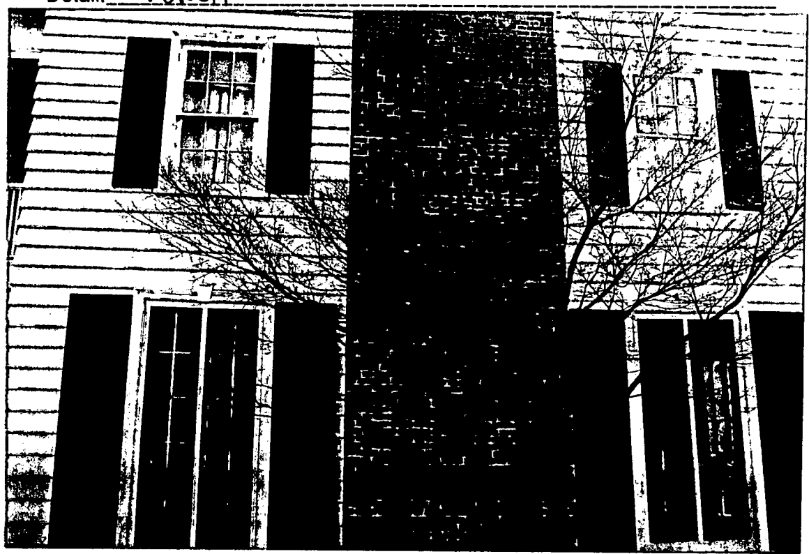
Detail: WEST FACADE
