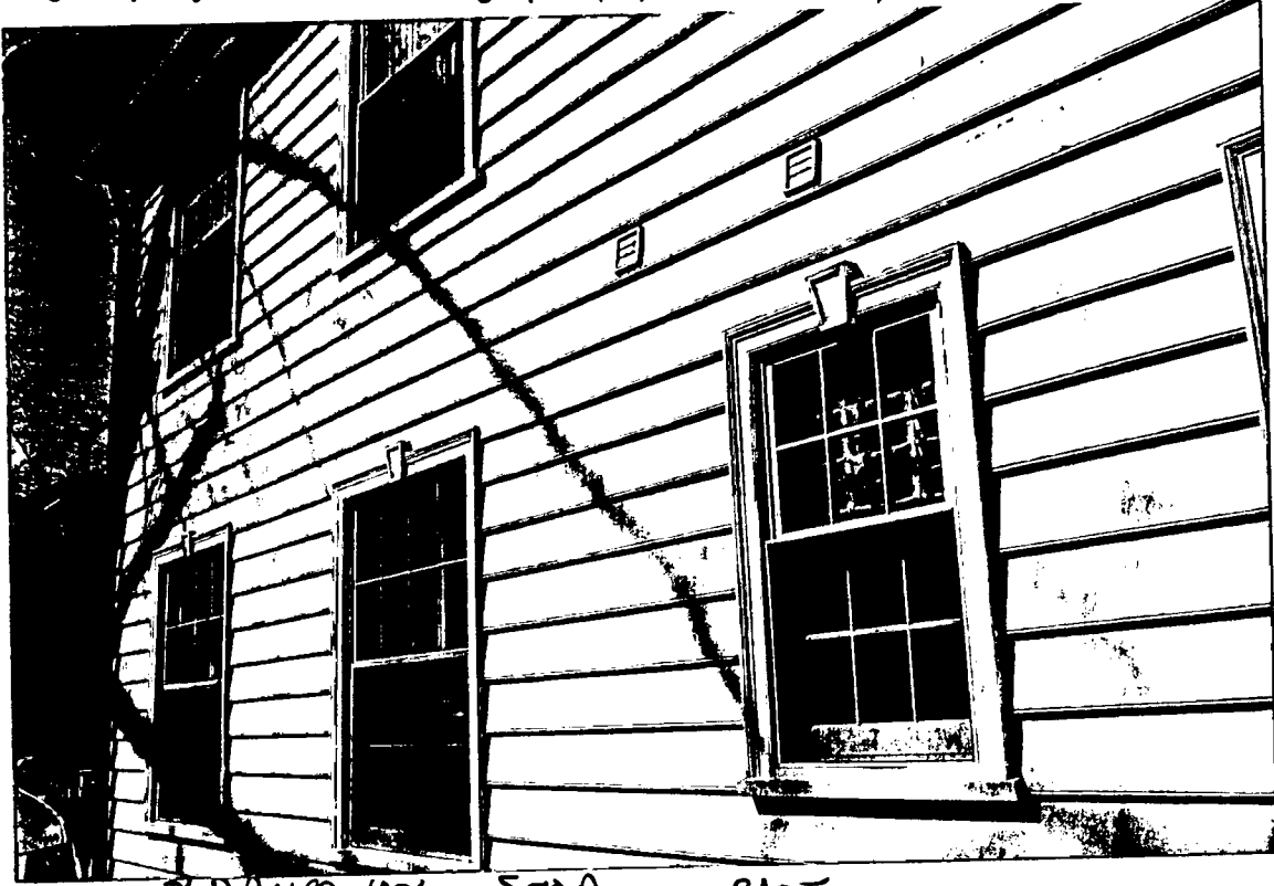
Detail: B DRIVEWAY SIDE EAST
