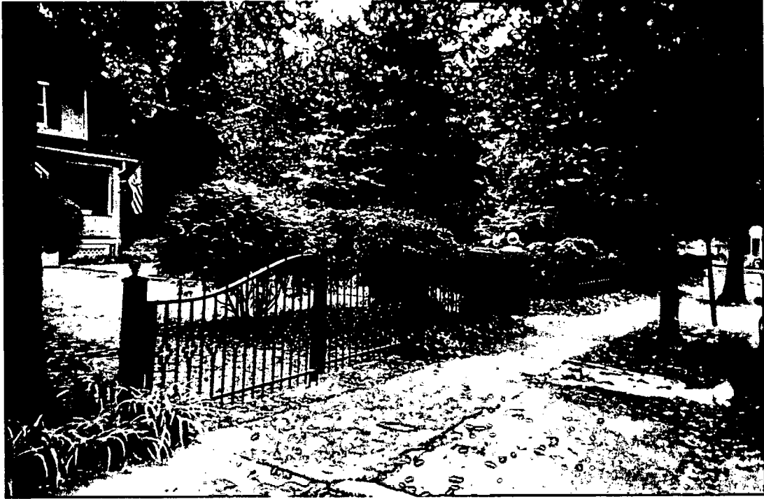
Detail: existing fence @ front of drive way
