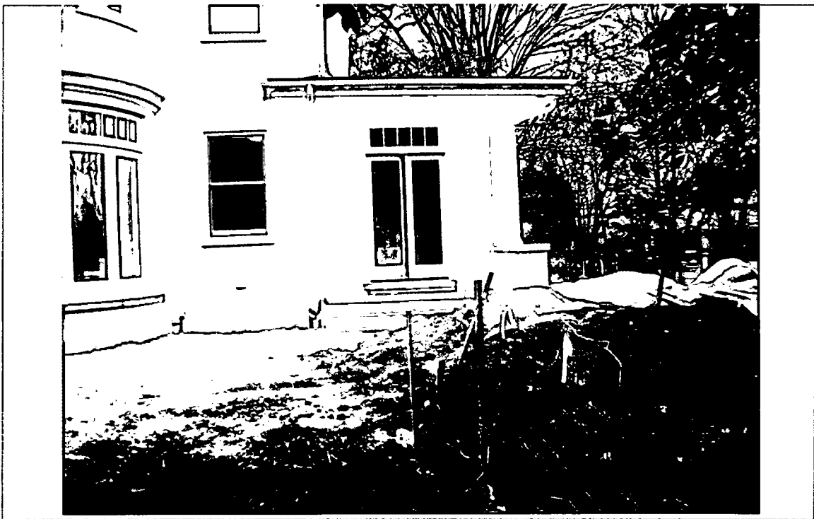
Detail: 8. View from North property line
