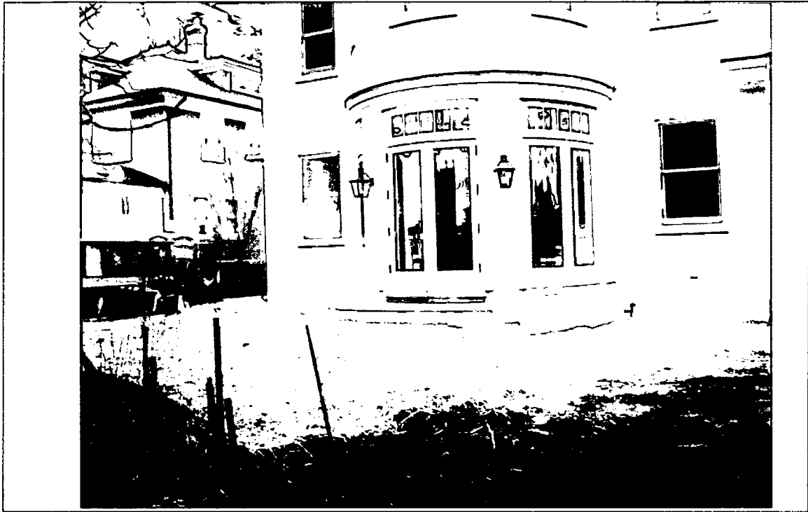
Detail: 7. View from North property line
