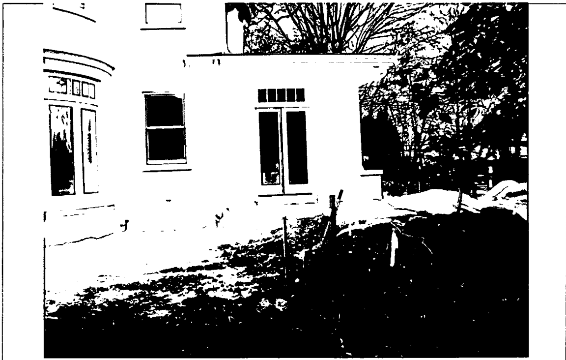
Detail: 8. View from North property line
