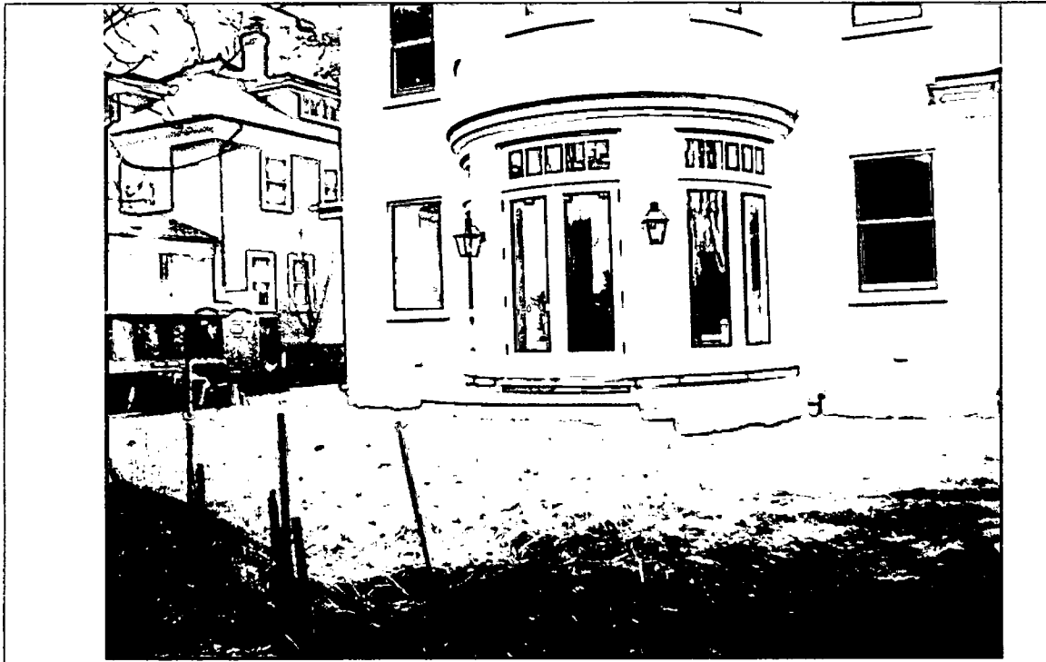
Detail: 7. View from North property line
