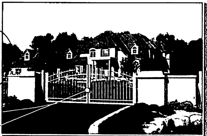
ARCHED DRIVE GATE WITH HIDE CONCEALED GATE OPENER
