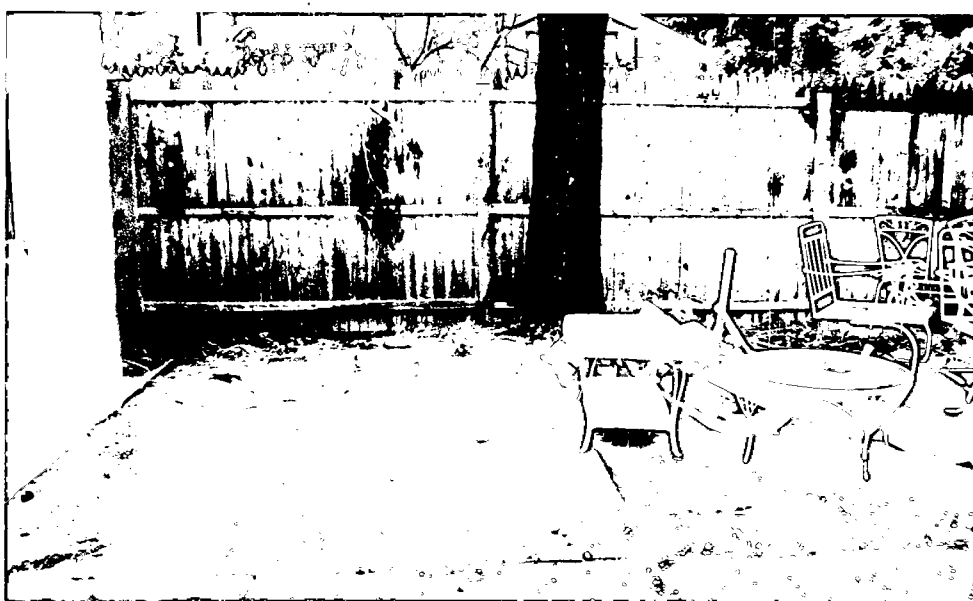
PHOTO OF HOMEOWNER'S PROPERTY WHERE WALL ON OTHER SIDE IS DETERIORATING THE MOST
