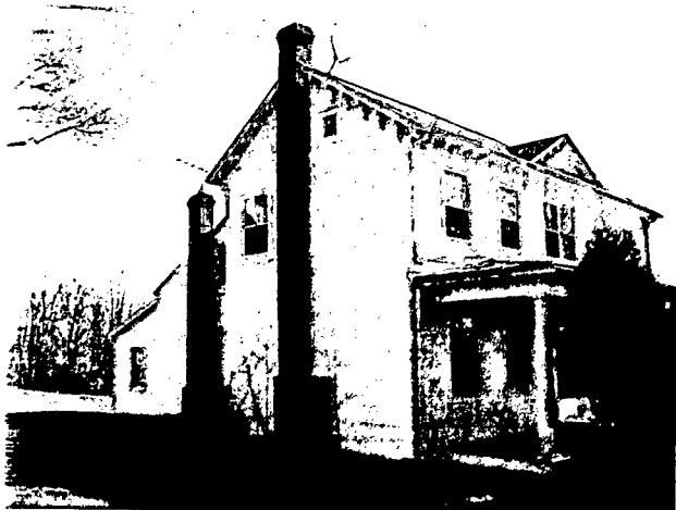
Image 10: North elevation showing where new period-type chimney made of salvaged brick and stone will replace rear chimney on log section of house. AC unit has already been moved.
