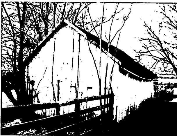
Image 16: Rear elevation of garage showing damage of volunteer tree growth prior to Parks' staff occupation of site.
