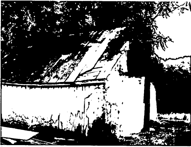
Image 15: Side elevation of garage showing deteriorating roof and subroofing and rotting wood wall planks.
