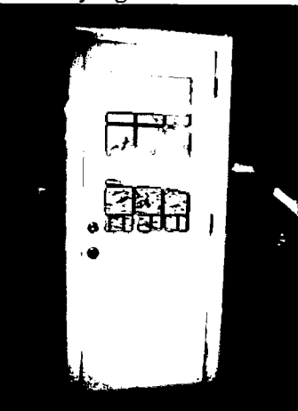
Image 6: Interior view of modern door located on the east (rear) elevation that will be replaced with a new, four-panel Greek Revival era-type door based on field investigation that such a door would have been added to the log structure in the Zeigler period (post 1854) and in the Greek Revival style.
