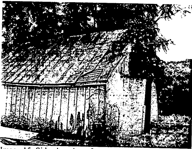
Image 15: Side elevation of garage showing deteriorating roof and subroofing and rotting wood wall planks.
