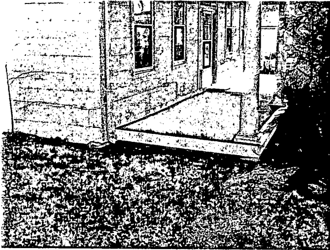
Image 4: The front porch (West elevation) where a new walkway with a shallow, ADA-compliant ramp will be constructed to allow for easier access to the house by all patrons.
