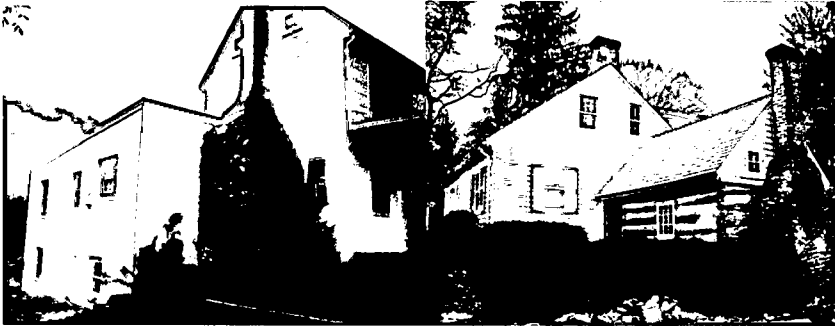
Images 11 and 12: Photos of similar exterior stone chimneys with brick stacks from structures of the first half of the 19 th century. Such stacks that will be recreated at the Zeigler House. Left: Perry Browning House (dendro dated to 1816); Right: the Josiah Henson Historic Site (log wing dendro dated to 1850).
