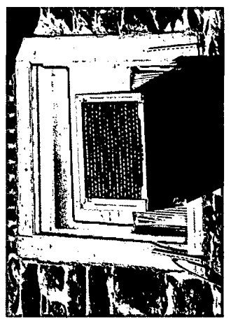
WINDOW 32 - FULL ELEVATION EXISTING AIR CONDITIONER & PLYWOOD FILLER PANEL ARE TO BE REMOVED. PREP FRAME OPENING AS REQUIRED & INSTALL A NEW WINDOW TO MATCH WINDOW #30 ADJACENT.
