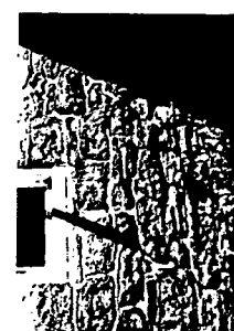
111 STONE DETAIL @ WINDOW # 11 - NO WORK REQUIRED AT STONE, REPOINT AND JOINTS AS NEEDED - WORK IS TO MATCH TYPE & COLOR OF EXISTING.
