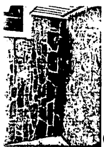
102 PARTIAL ELEVATION @ EAST END OF PORCH * REMOVE EXISTING STONE PORCH AND REPAIR AS NECESSARY TO MATCH TYPE & COLOR OF EXISTING. REPAIR AS NECESSARY TO MATCH TYPE & COLOR OF EXISTING. REPAIR AS NECESSARY TO MATCH TYPE & COLOR OF EXISTING. REPAIR AS NECESSARY TO MATCH TYPE & COLOR OF EXISTING.
