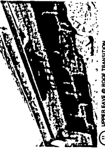
107 UPPER LEAVE @ ROOF TRANSITION - PATON & BEANE LISTING BOARD 1 & 2, AS REFERRED TO IN ARCHITECTURAL SPECIFICATIONS & EXISTING OVERHANG & FINISH BOARDING TO BE RESTORED, FINISHED & PAINTED TO MATCH EXISTING LIGHT FIXTURES & PROVIDE (2) NEW FIXTURES. (1) FOR EACH SIDE OF DOOR, NEW FIXTURES SHALL MATCH THE PROFILE OF THE HOUSE.
