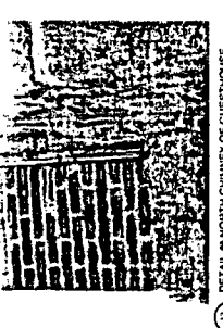
DETAIL @ NORTH CHIMNEY & GUESTHOUSE EXISTING BRICK CHIMNEY TO BE REPAIRED. PATCH AS REPAIRS AS REQUIRED. REMOVE OLD ANTENNA & PATCH INHOMOGENEOUS AS NEEDED.
