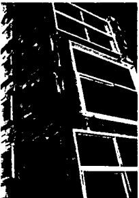
1.03 ROOF EDGE & WINDOW ADDITION EXISTING CEDAR WOOD FRAME WINDOW TO BE REPLACED BY FRAME OF PALACE WINDOW WITH NEW EXTERIOR AND INTERIOR FINISHES. WINDOW TO BE SET INTO EXISTING WALL WITH NEW FINISHES. WINDOW TO BE SET INTO EXISTING WALL WITH NEW FINISHES.
