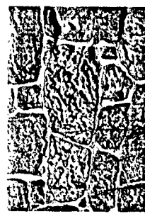
STONE DETAIL NO WORK REQUIRED - STONE REPORTING AND JOINTS AS NEEDED - MATCH TYPE & COLOR OF EXISTING.
