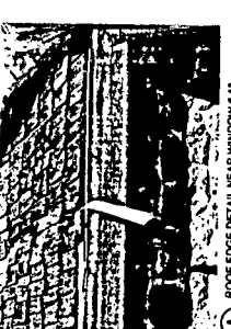
106 ROOF EDGE DETAIL NEAR WINDOW # 11 - PATON & BEANE LISTING BOARD 1 & 2, AS REFERRED TO IN ARCHITECTURAL SPECIFICATIONS & EXISTING OVERHANG & FINISH BOARDING TO BE RESTORED, FINISHED & PAINTED TO MATCH EXISTING LIGHT FIXTURES & PROVIDE (2) NEW FIXTURES. (1) FOR EACH SIDE OF DOOR, NEW FIXTURES SHALL MATCH THE PROFILE OF THE HOUSE.
