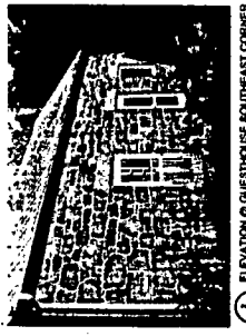
ELEVATION & GUESTHOUSE SOUTHWEST CORNER EXISTING METAL ROOFING TO BE REMOVED. PATCH AS REPAIRS AS REQUIRED. REMOVE OLD ANTENNA & PATCH INHOMOGENEOUS AS NEEDED. REMOVE OLD ANTENNA & PATCH INHOMOGENEOUS AS NEEDED.
