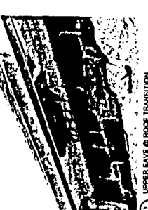
107 UPPER LEAVE @ ROOF TRANSITION - PATON & BEANE LISTING BOARD 1 & 2, AS REFERRED TO IN ARCHITECTURAL SPECIFICATIONS & EXISTING OVERHANG & FINISH BOARDING TO BE RESTORED, FINISHED & PAINTED TO MATCH EXISTING LIGHT FIXTURES & PROVIDE (2) NEW FIXTURES. (1) FOR EACH SIDE OF DOOR, NEW FIXTURES SHALL MATCH THE PROFILE OF THE HOUSE.
