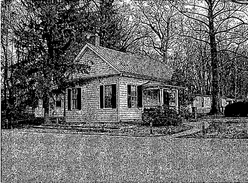
Current view of the Community House from the southwest parking lot showing south and west facades. The recessed east wing of the building visible in the photo will be demolished (built 1978 and 1985). The back low-slope addition on the north side will remain. The visible corner of the graveyard fence will be chamfered (Two stone fence posts will replace the one.) The tulip poplar will be removed.
