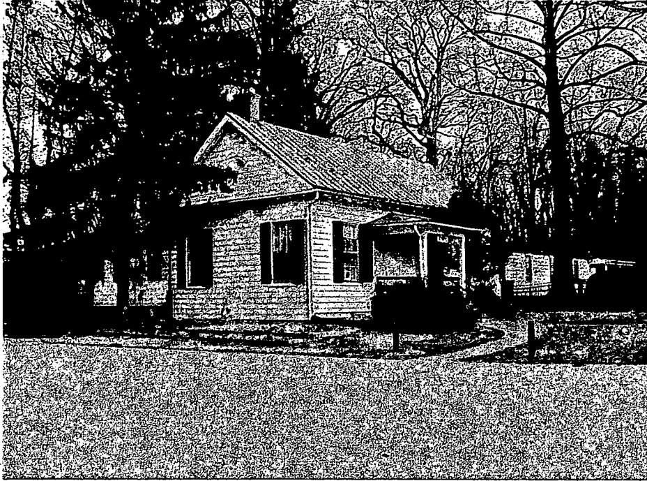
Current view of the Community House from the southwest parking lot showing south and west facades. The recessed east wing of the building visible in the photo will be demolished (built 1978 and 1985). The back low-slope addition on the north side will remain. The visible corner of the graveyard fence will be chamfered (Two stone fence posts will replace the one.) The tulip poplar will be removed.
