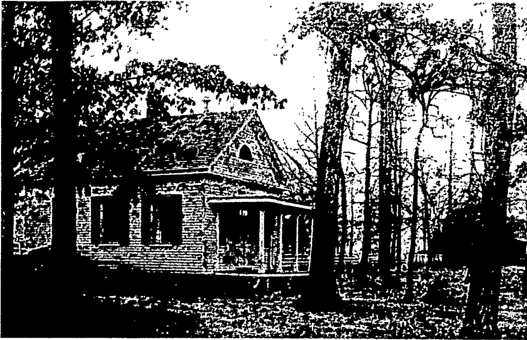
Historic photo of the Lyceum taken from the northwest. The meeting house is visible to the south. If the original lap siding is intact, it will be restored.
