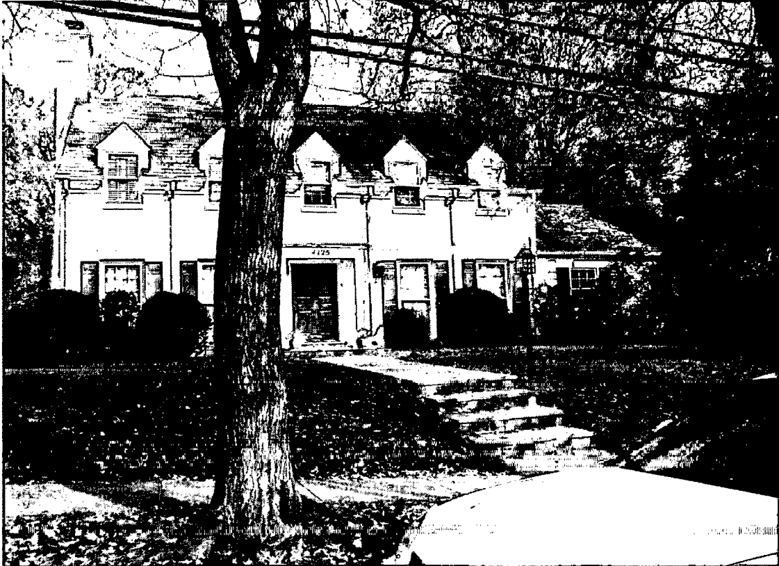
Fig. 9: 4725 Dorset Ave - Attached two-car garage (front view)
