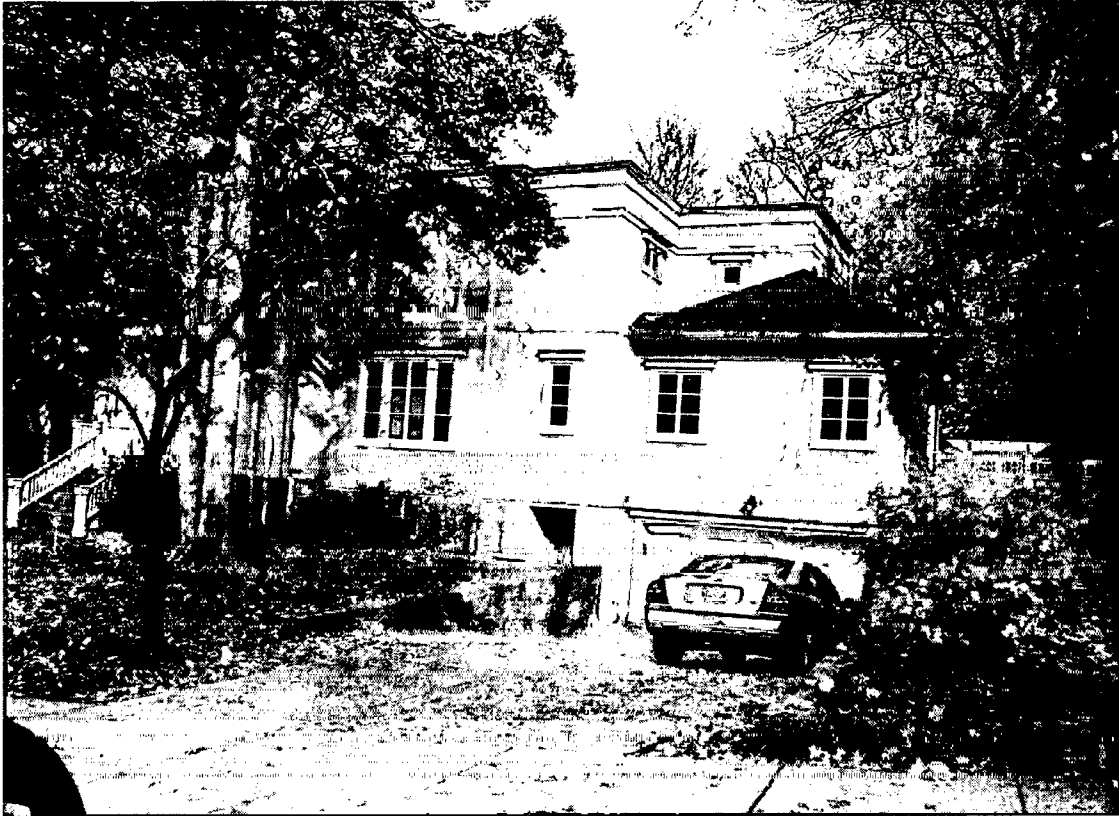
Fig. 13: 4901 Dorset Ave - Attached cellar level two-car garage facing street
