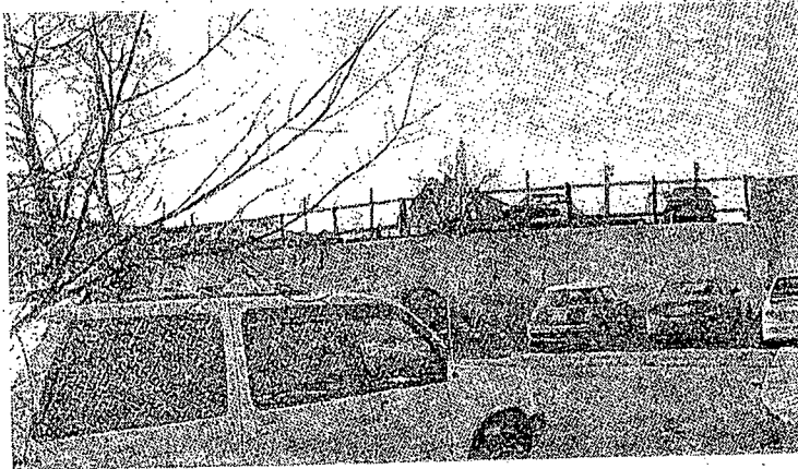
VIEW 4 Looking North from Property Interior
