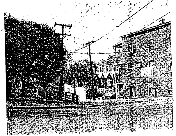
VIEW 3 Looking South along Westmoreland Ave
