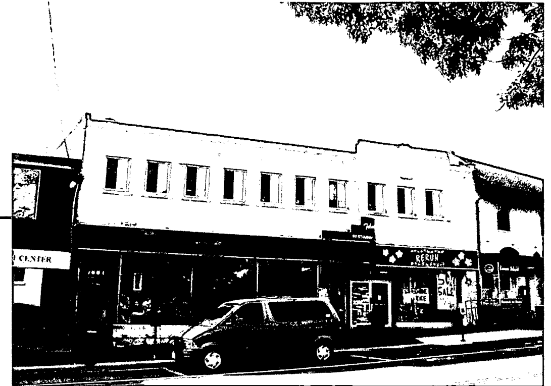
HISTORIC STOREFRONT RESTORATION
