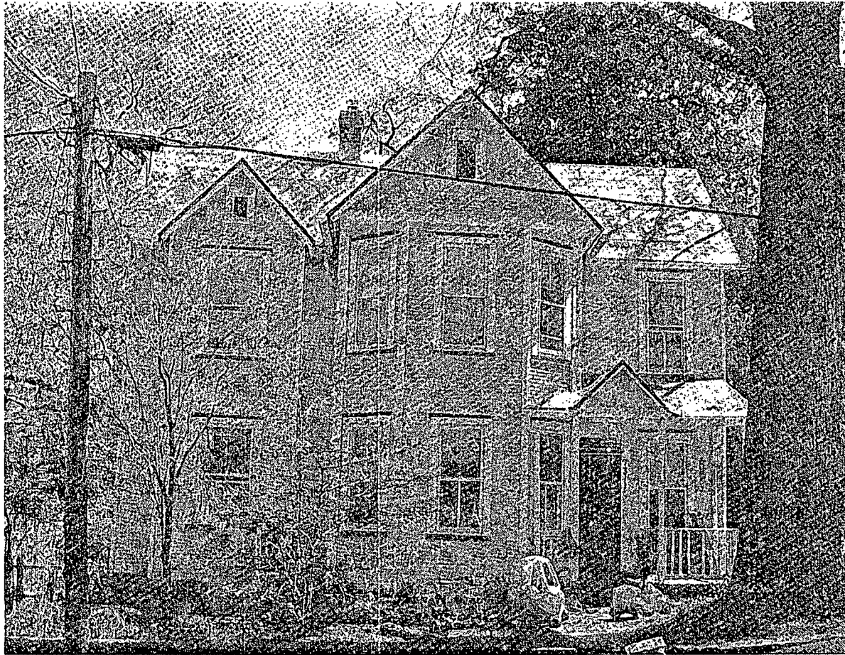
Northwest Elevation (Street Elevation) of House
