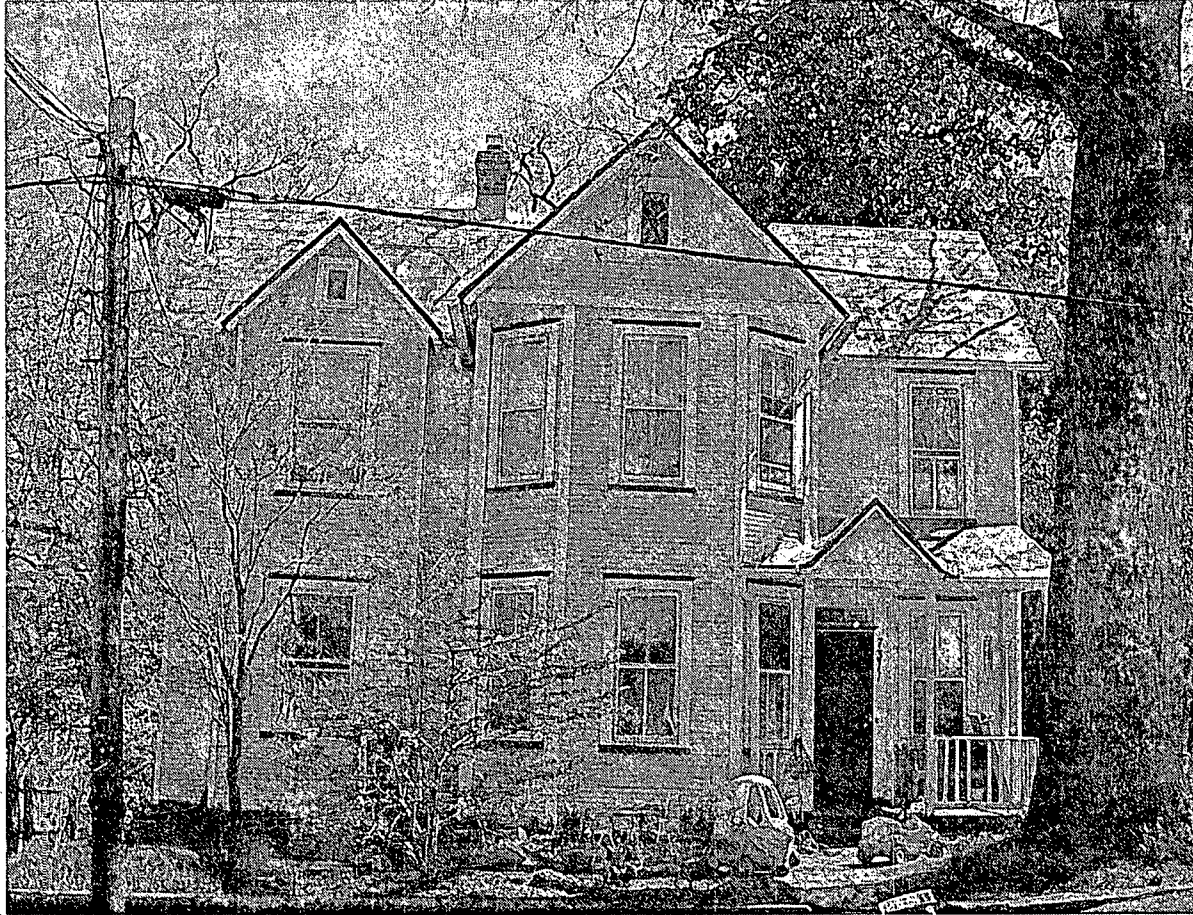
Northwest Elevation (Street Elevation) of House
