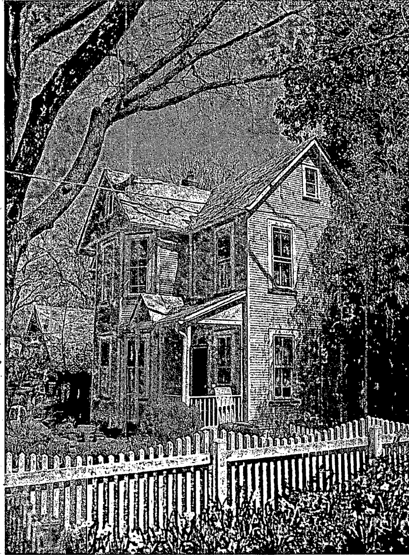
View of West corner of house
