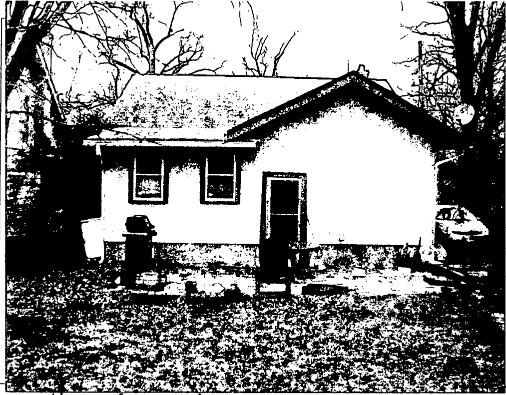
Detail: Rear of Property
