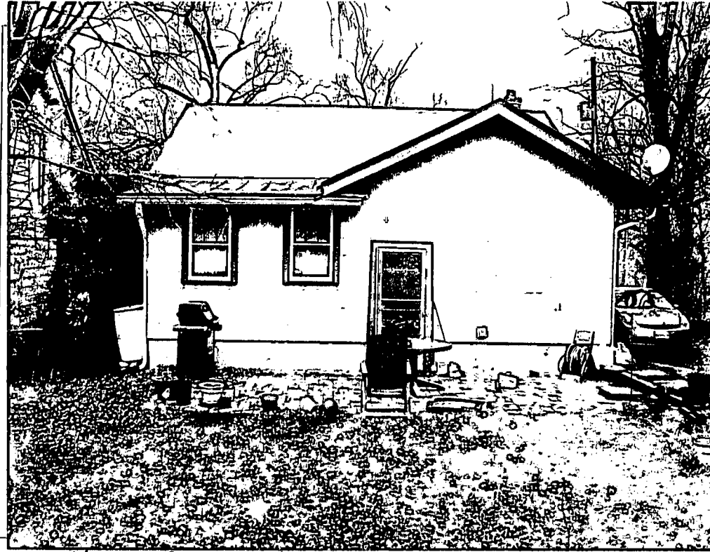
Detail: Kear of Property
