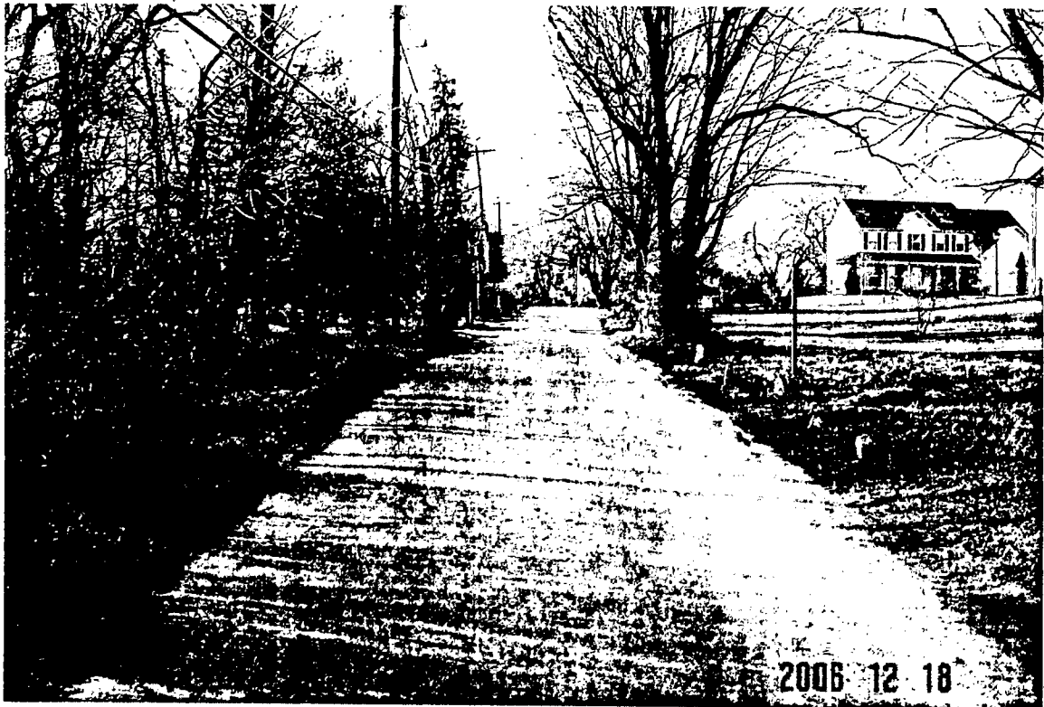
FACING SOUTH ON OAK HILL ROAD
