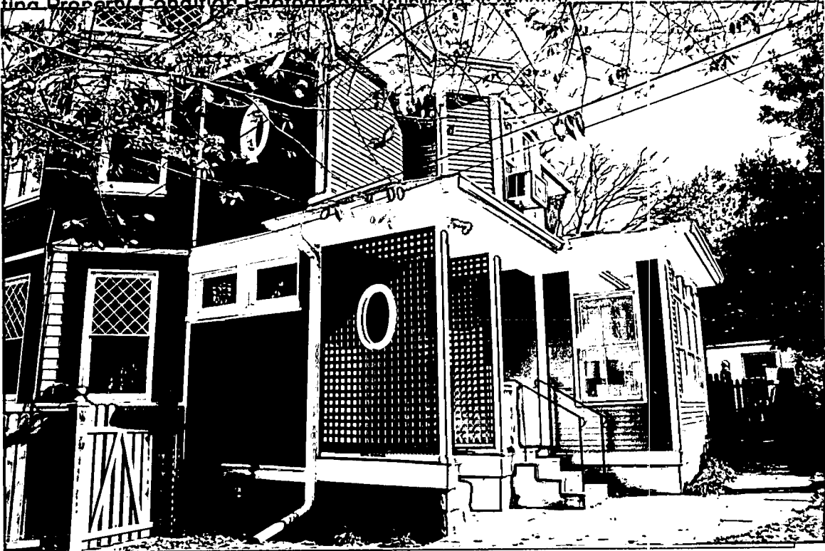
Detail: WEST VIEW FROM SIDE YARD REAR
