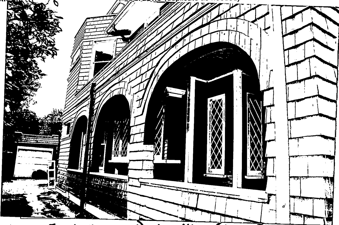
Detail: EAST VIEW - DRIVEWAY SIDE FROM FRONT
