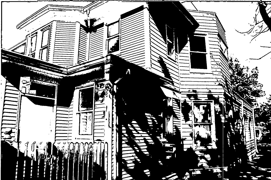
Detail: EAST VIEW - DRIVEWAY SIDE FROM REAR
