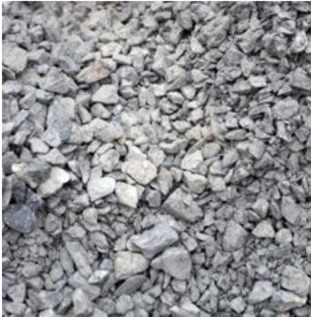
21A Gravel (Crusher Run) installed 8" deep (2x 4" lifts)
