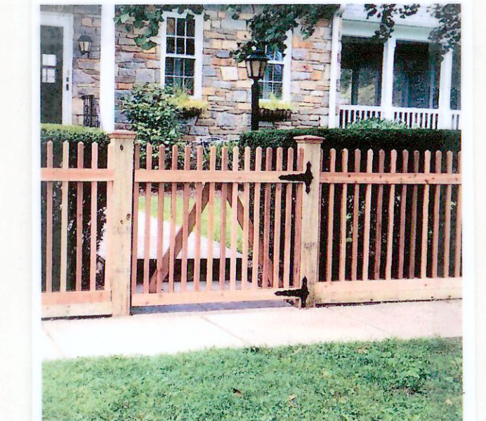
Picket Style Fencing and Gate 5ft. high
