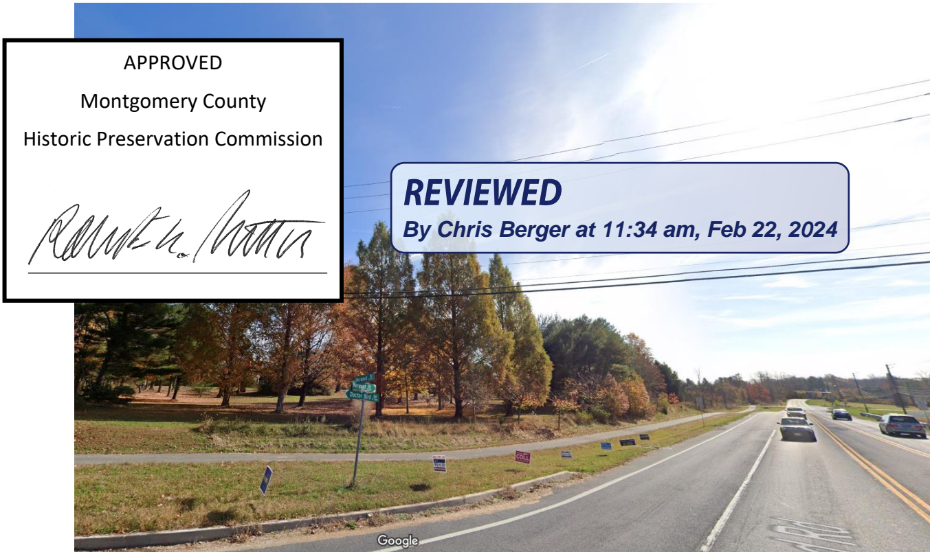
Photo 2: Norwood property and SUP, looking southeast from intersection of Norwood and Dr. Bird Roads (Google Street View, November 2022)
