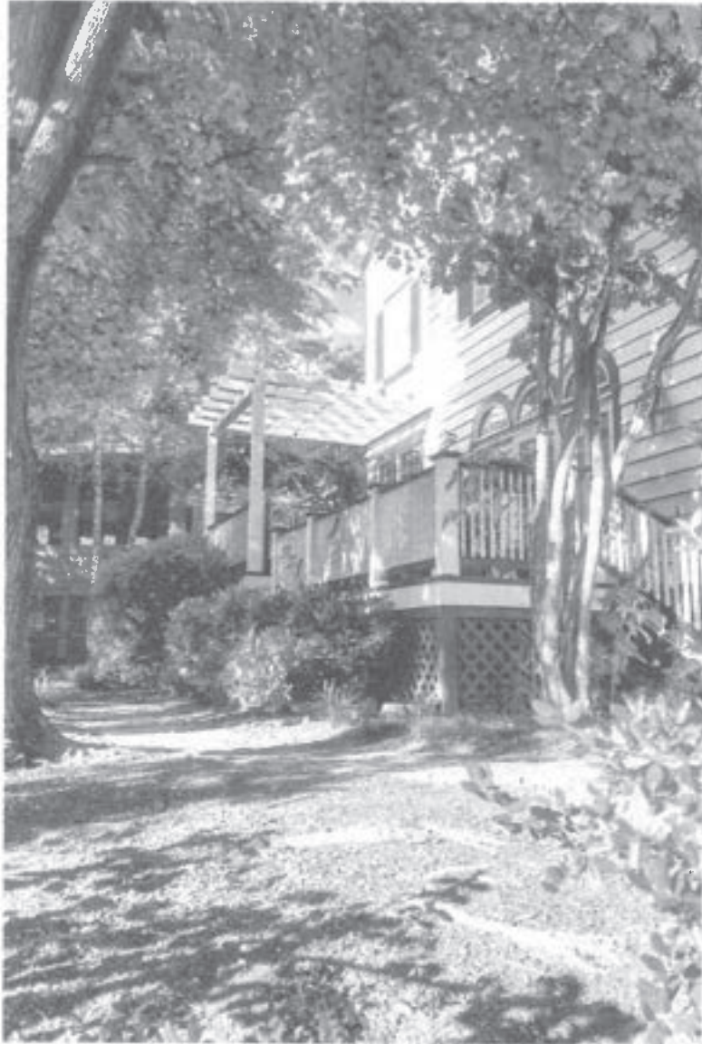
NORTH ELEVATION OF DECK - Dec. 2023
