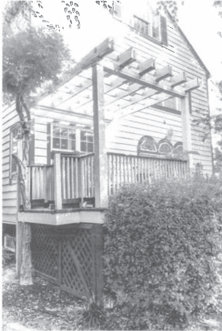
South Elevation of Deck - Dec. 2023
