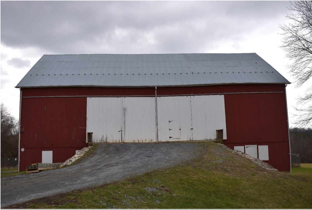
Bank Barn, existing conditions
