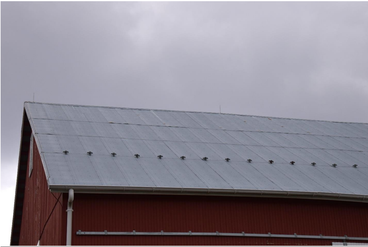
(Existing lightning system to be put back)
