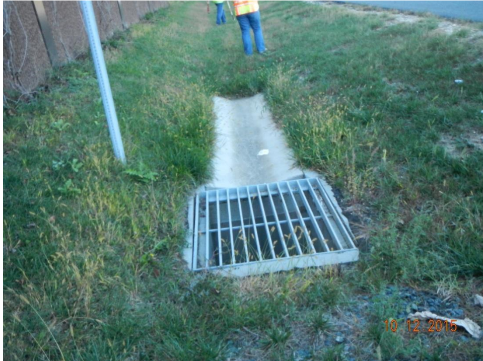
Photo 1: Example of a K inlet with concrete gutter. Note that the gutter is not used for all K inlets and where it is used, it may be used on both sides.
