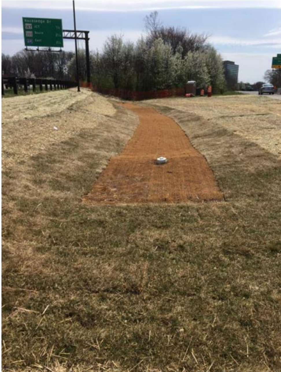
Photo 5: Image of bioswale similar to what is proposed on the Red Door Store property (RK&K photo)
