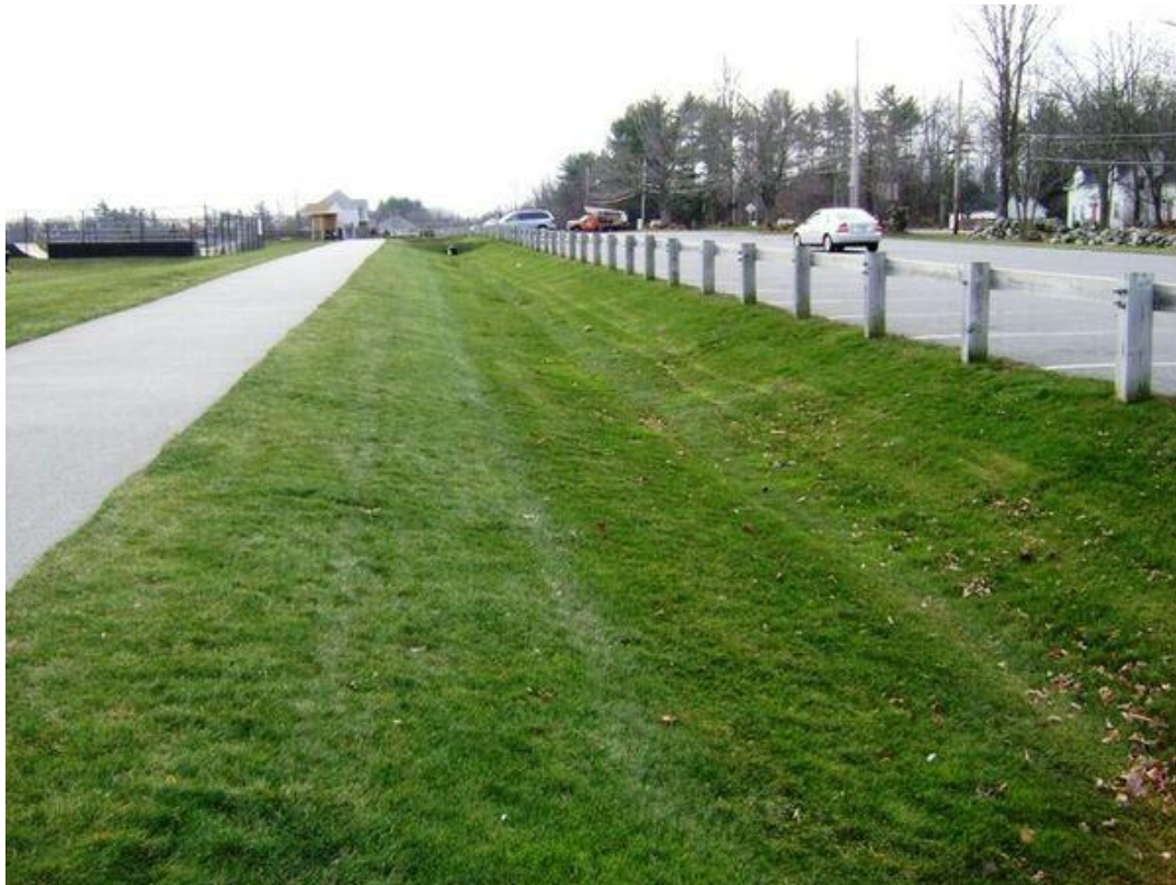
Photo 4: Image of bioswale similar to what is proposed on the Red Door Store property (RKK Photo)
