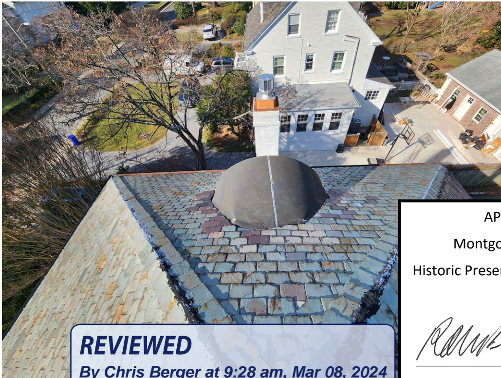
After - west side dormer:
