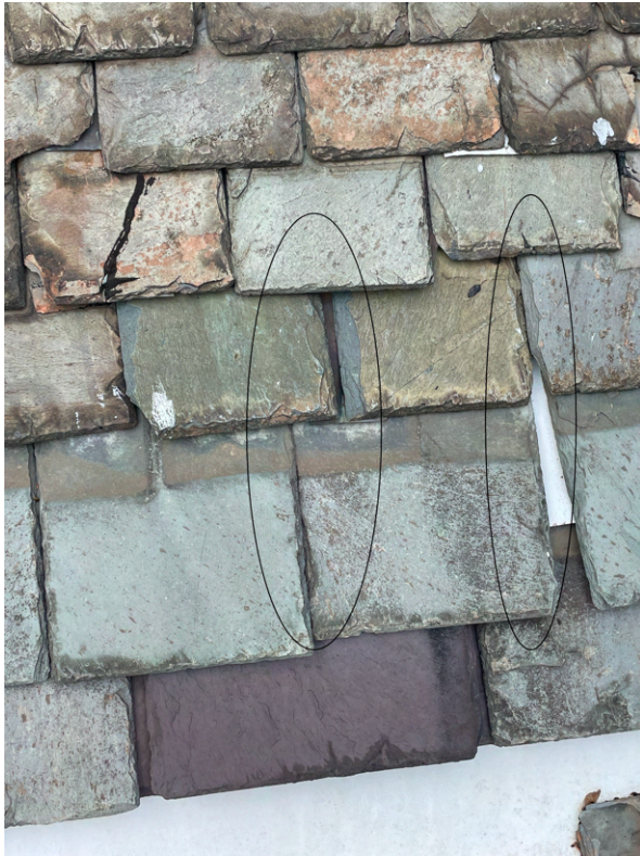
Before - east side tiles to reinstall:
