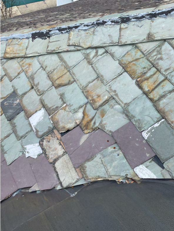
Before - west side dormer:
