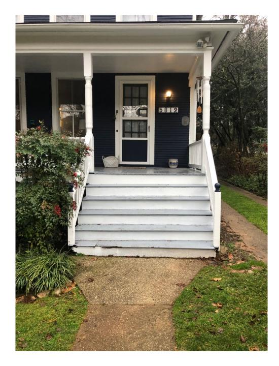
Zoomed in picture of stairs. Deteriorated bottom step visible. Rotted and missing wood seen on bottom step.
