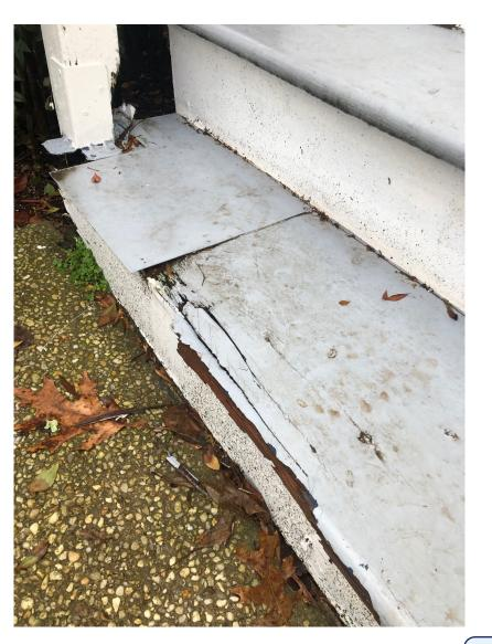
Rotted bottom step. 1 ft by 1 ft metal cover – installed by former owner – visible.
