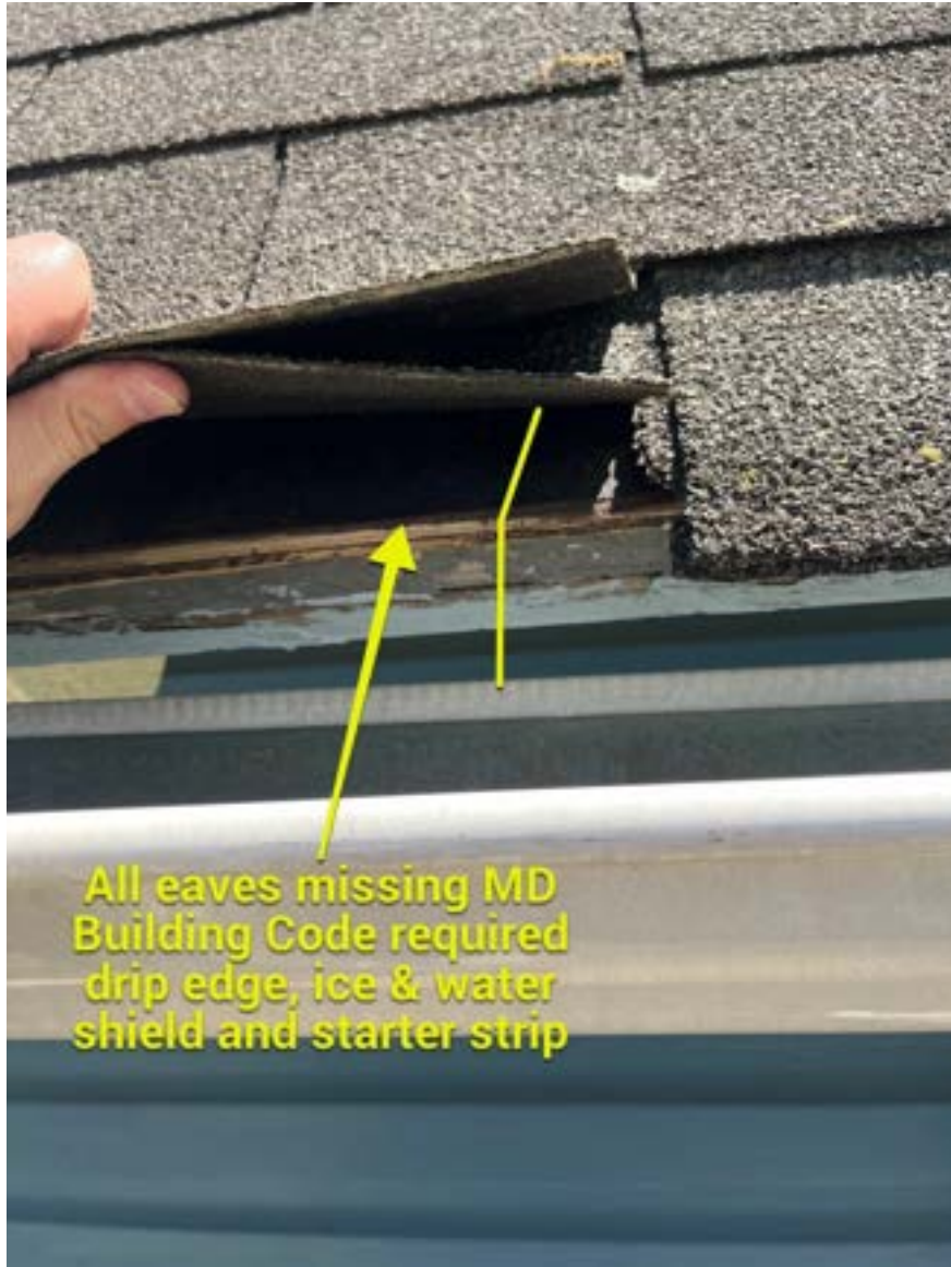
31. Close up of roof edge
