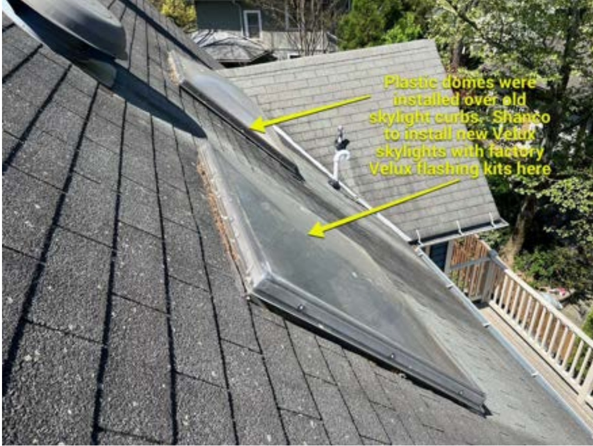
23. Upper side roof showing skylights
