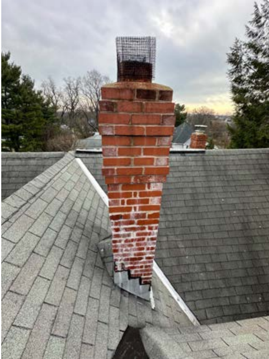
13. Middle chimney, view from back of house
