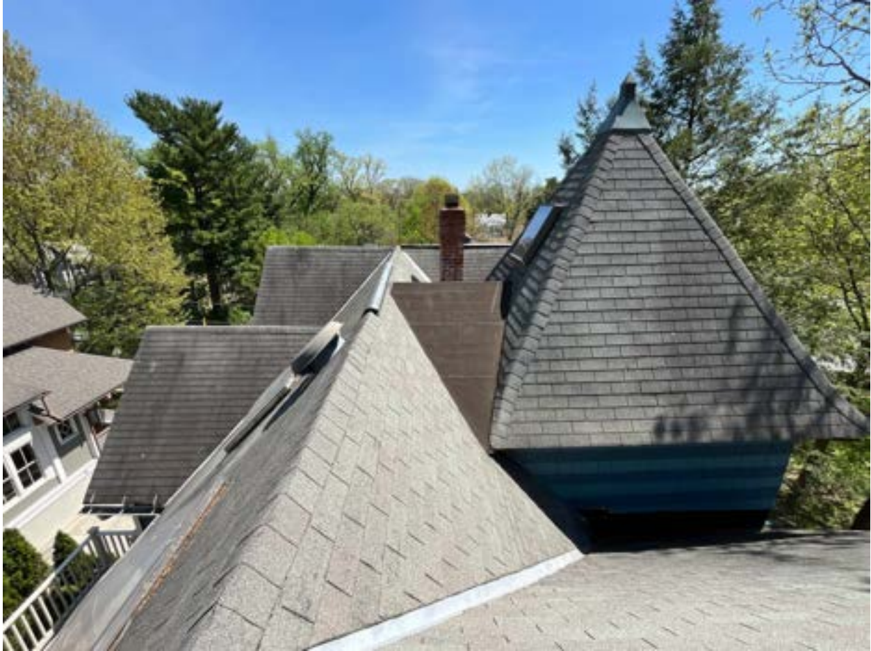
30. View of roof from back of house
