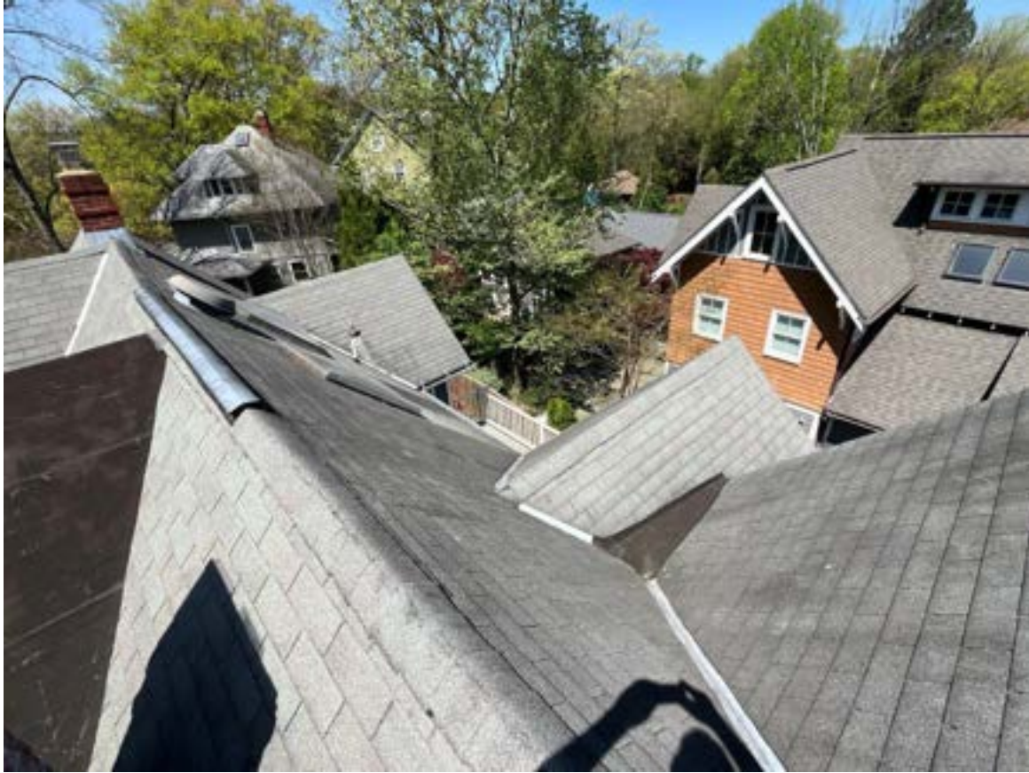
25. Upper roof view
