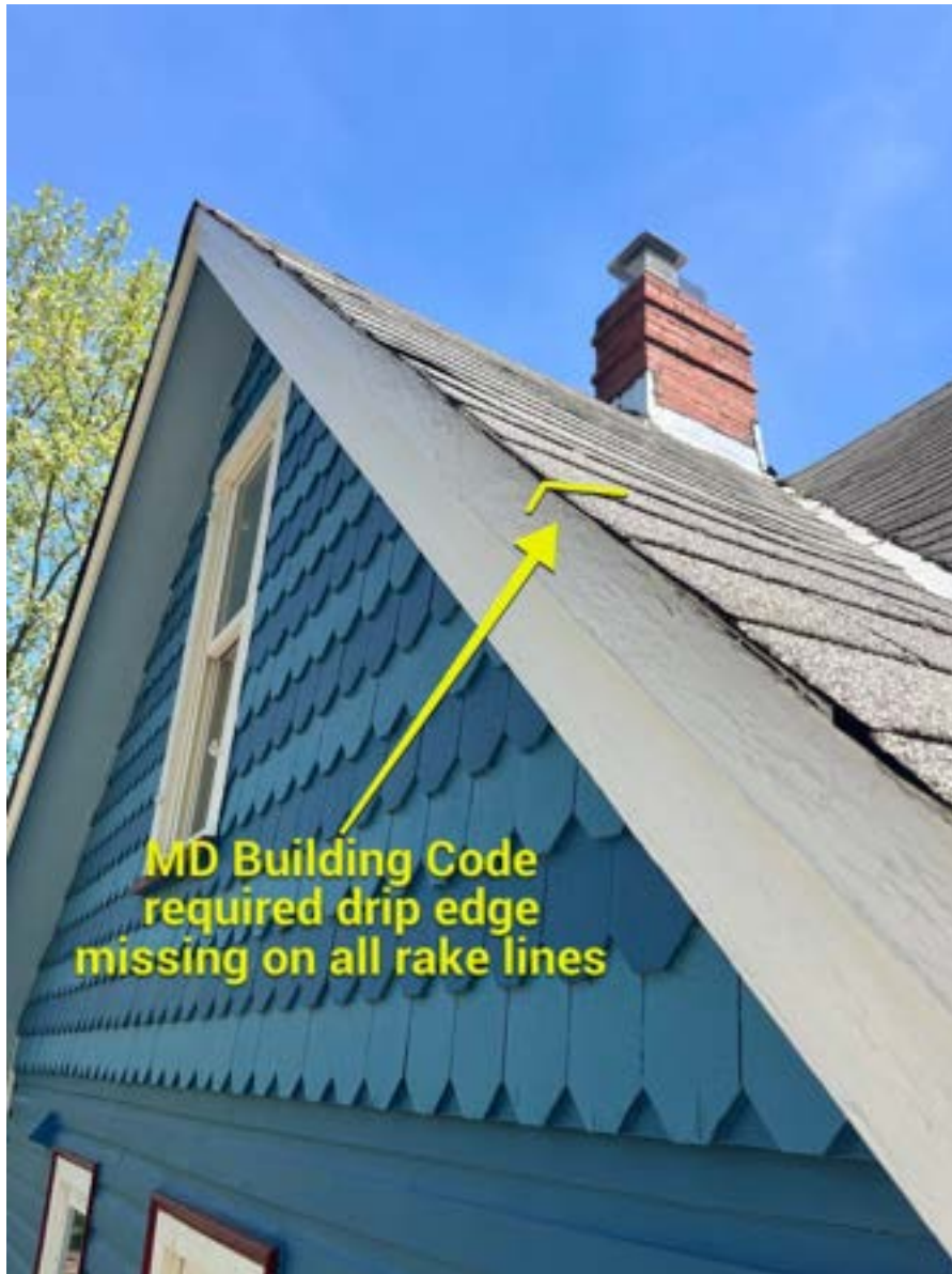
21. Roof at back of house
