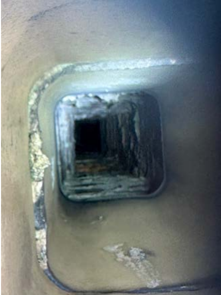
16. Chimney interior view
