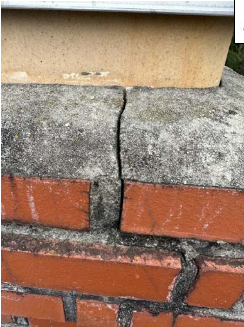
6. Front chimney (orphan chimney) close up
