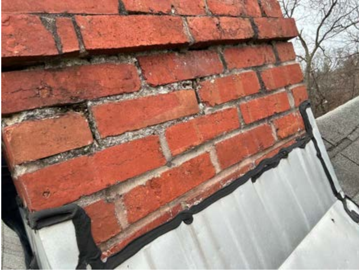
19. Back chimney, close up
