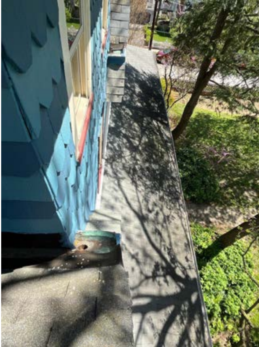
29. Side porch roof view
