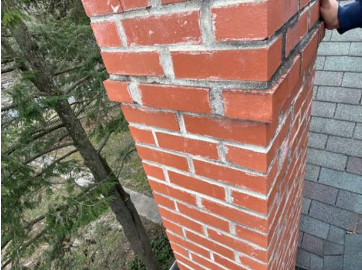
5. Front chimney (orphan chimney)
