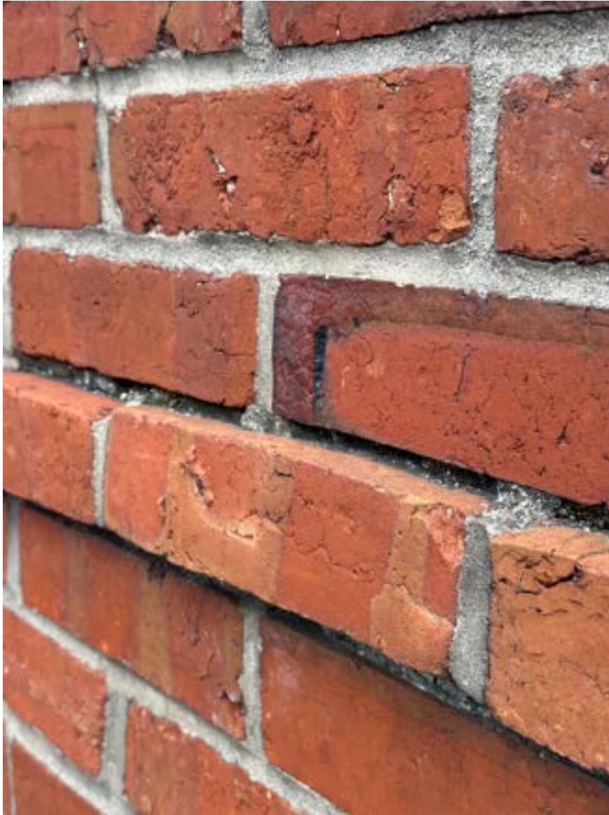
20. Back chimney, close up
