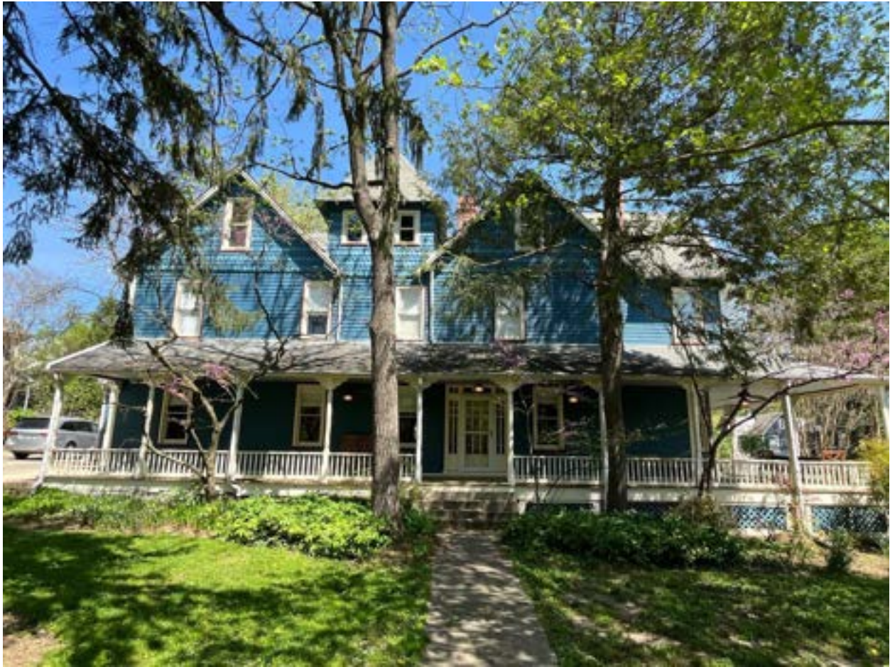
3. Side porch view
