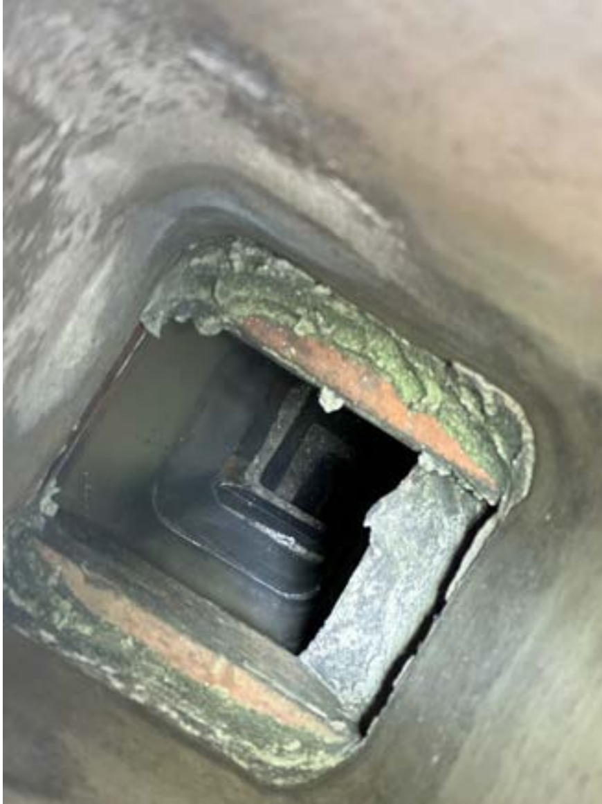
15. Chimney interior view
