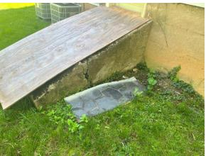
Note: temporary plywood sheet recently set in place to deflect rain in an attempt to mitigate on-going water infiltration issues.
